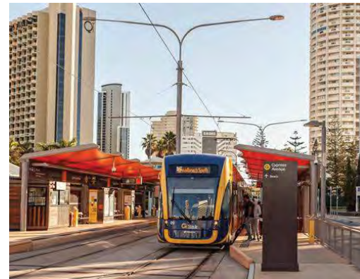
Cypress Avenue Light Rail Station, Gold Coast
