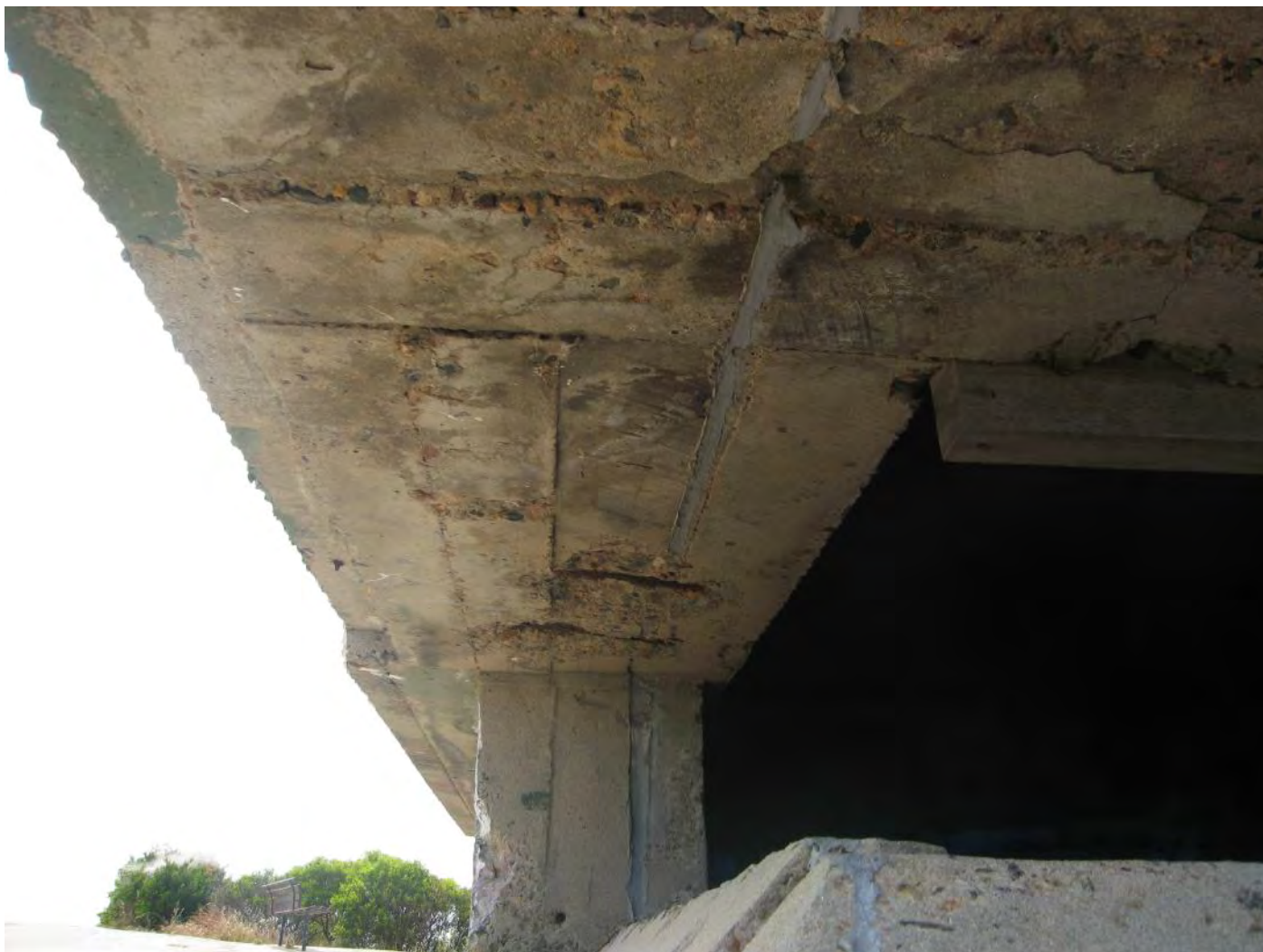
Figure 61: Underside of Concrete Overhang to Observation Opening
