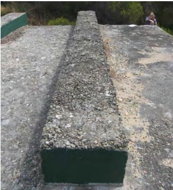
Figure 82: Operations Bunker – Reinforced concrete roof beam
