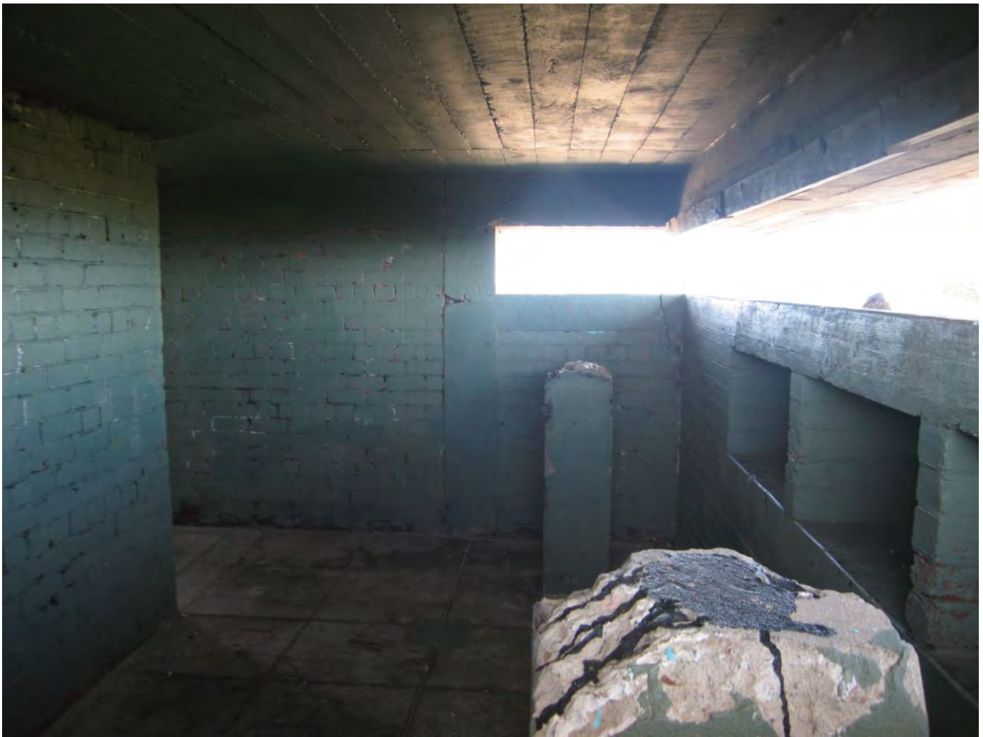
Figure 67: Ground level interior
