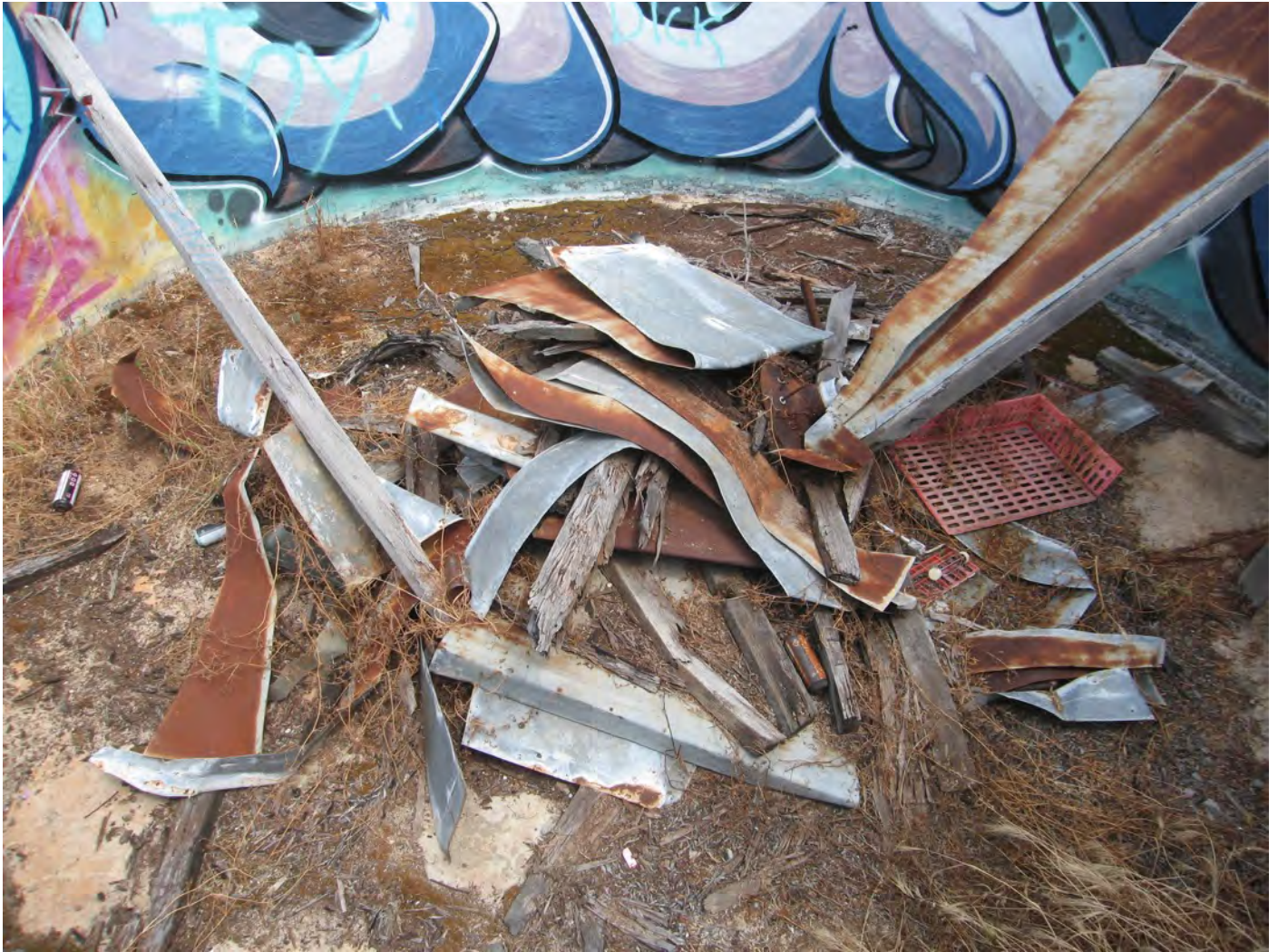
Figure 155: Water Tank – interior of water tank with remnant roofing fabric
