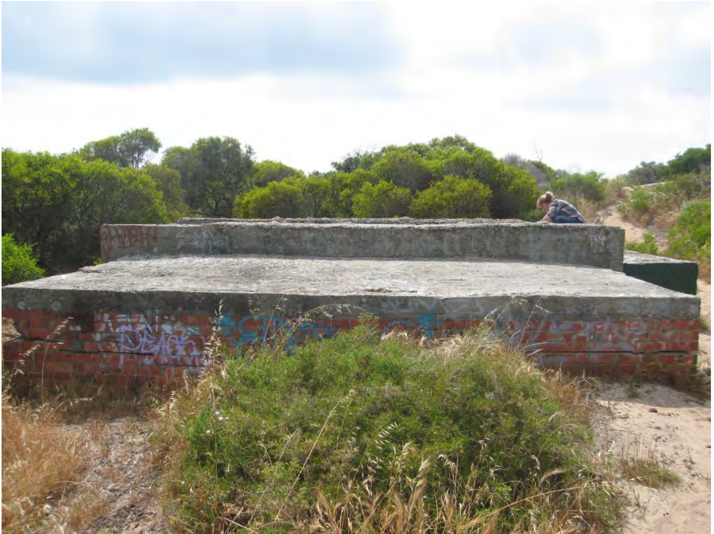
Figure 84: Operations Bunker – west elevation
