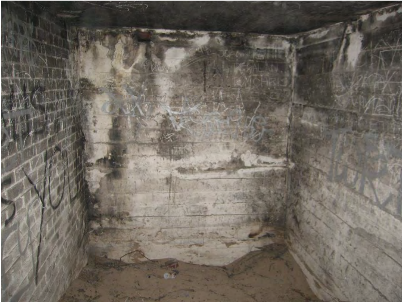
Figure 122: Ammunition Bunker – Room 1
