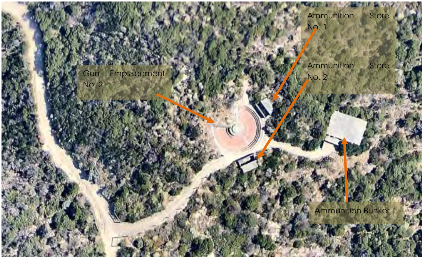
Figure 140: Gun Emplacement No. 2 and Ammunition Bunker Courtesy Nearmap, 2015
