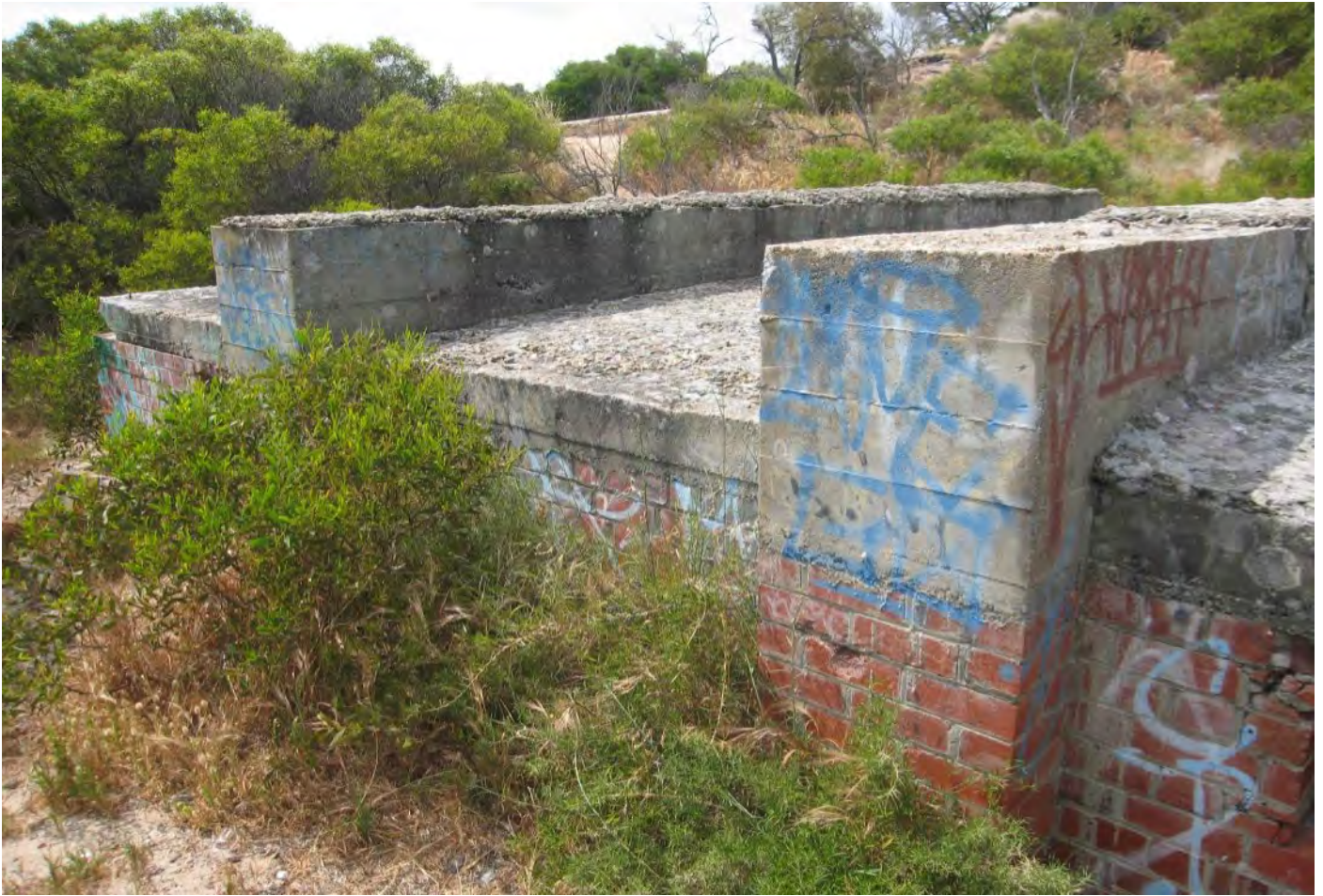
Figure 81: Operations Bunker – North wall
