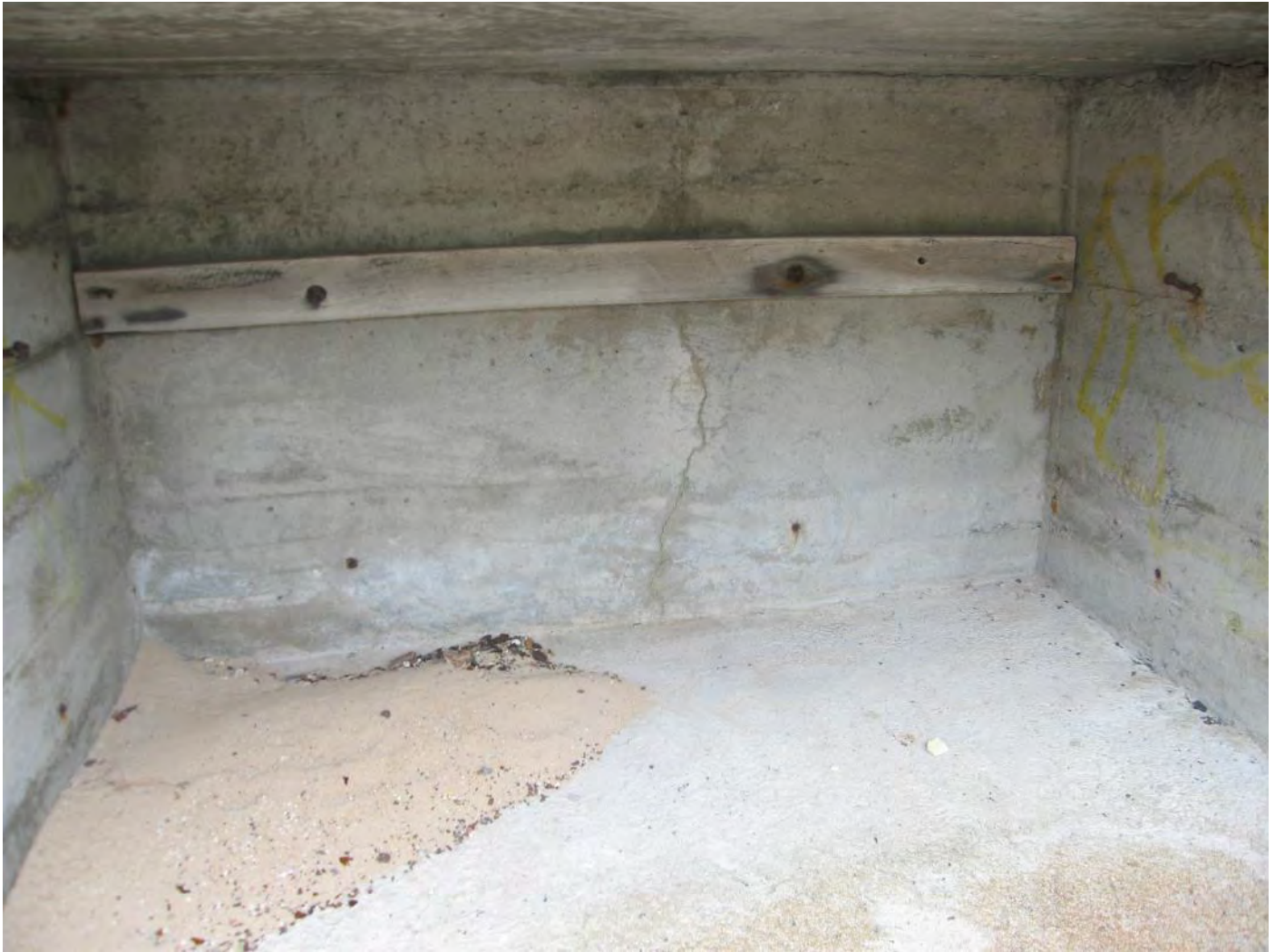
Figure 109: Gun Emplacement - Ammunition Store No. 1
