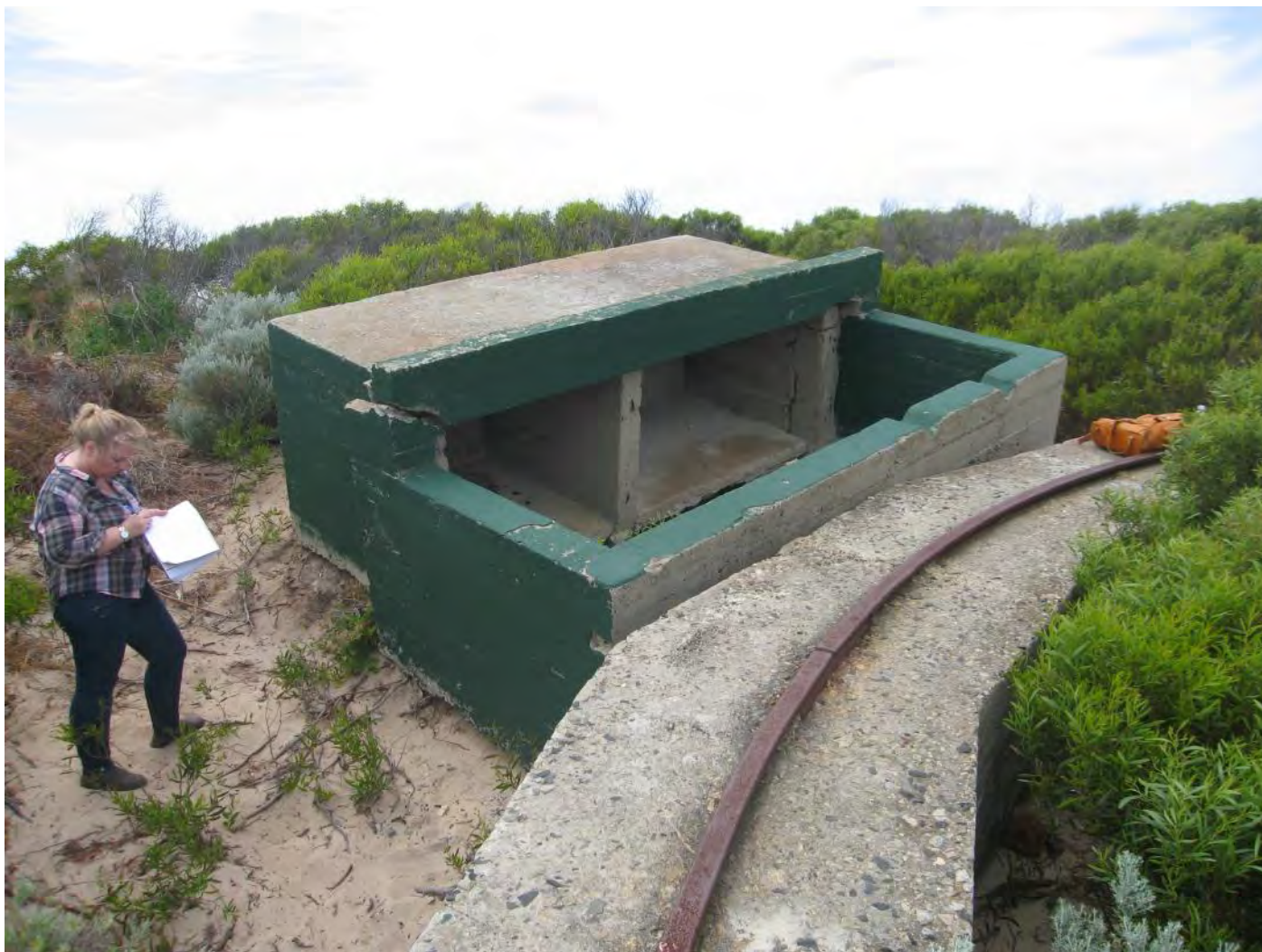
Figure 106: Gun Emplacement - Ammunition Store No. 1
