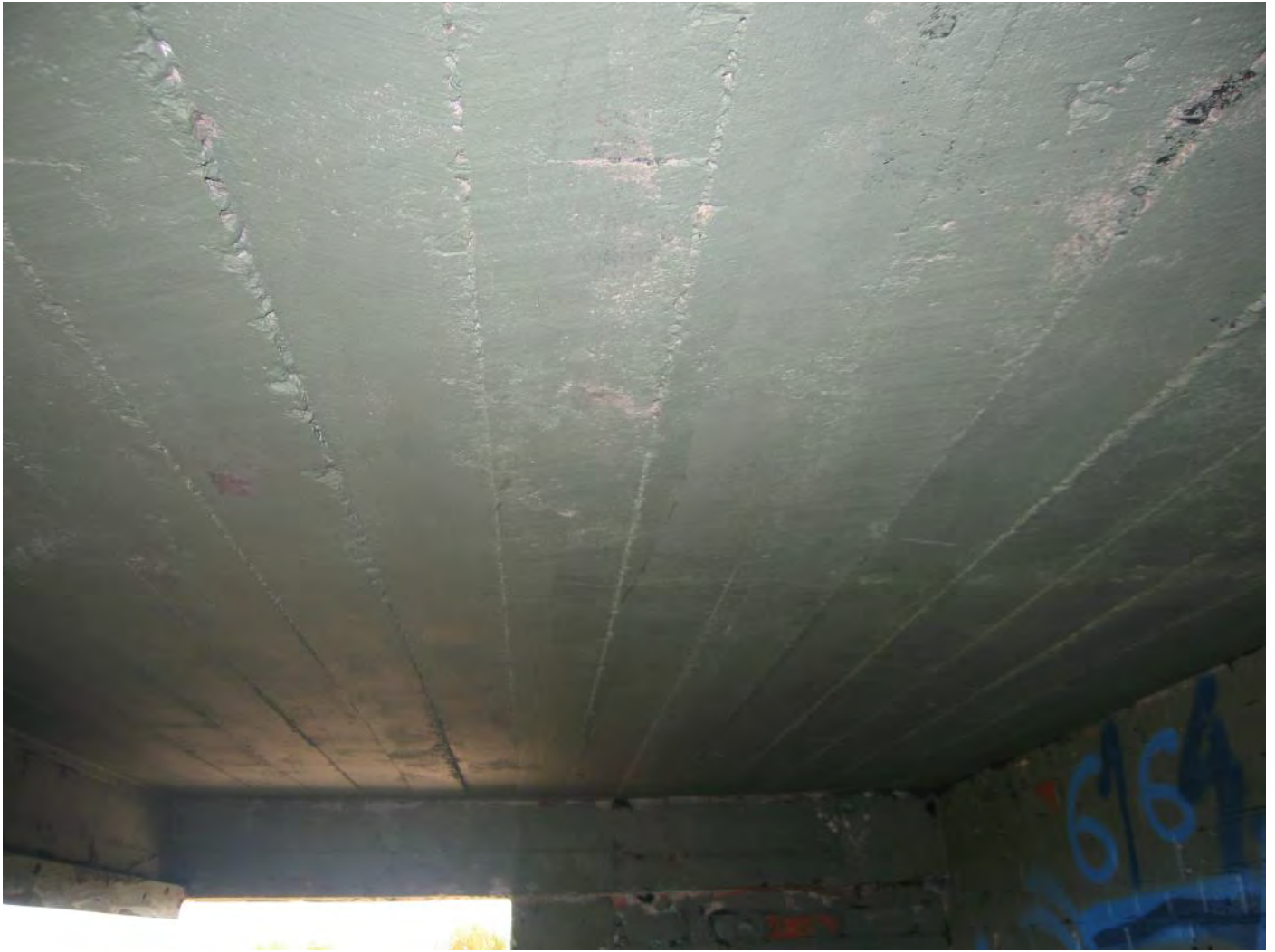
Figure 74: Concrete slab roof
