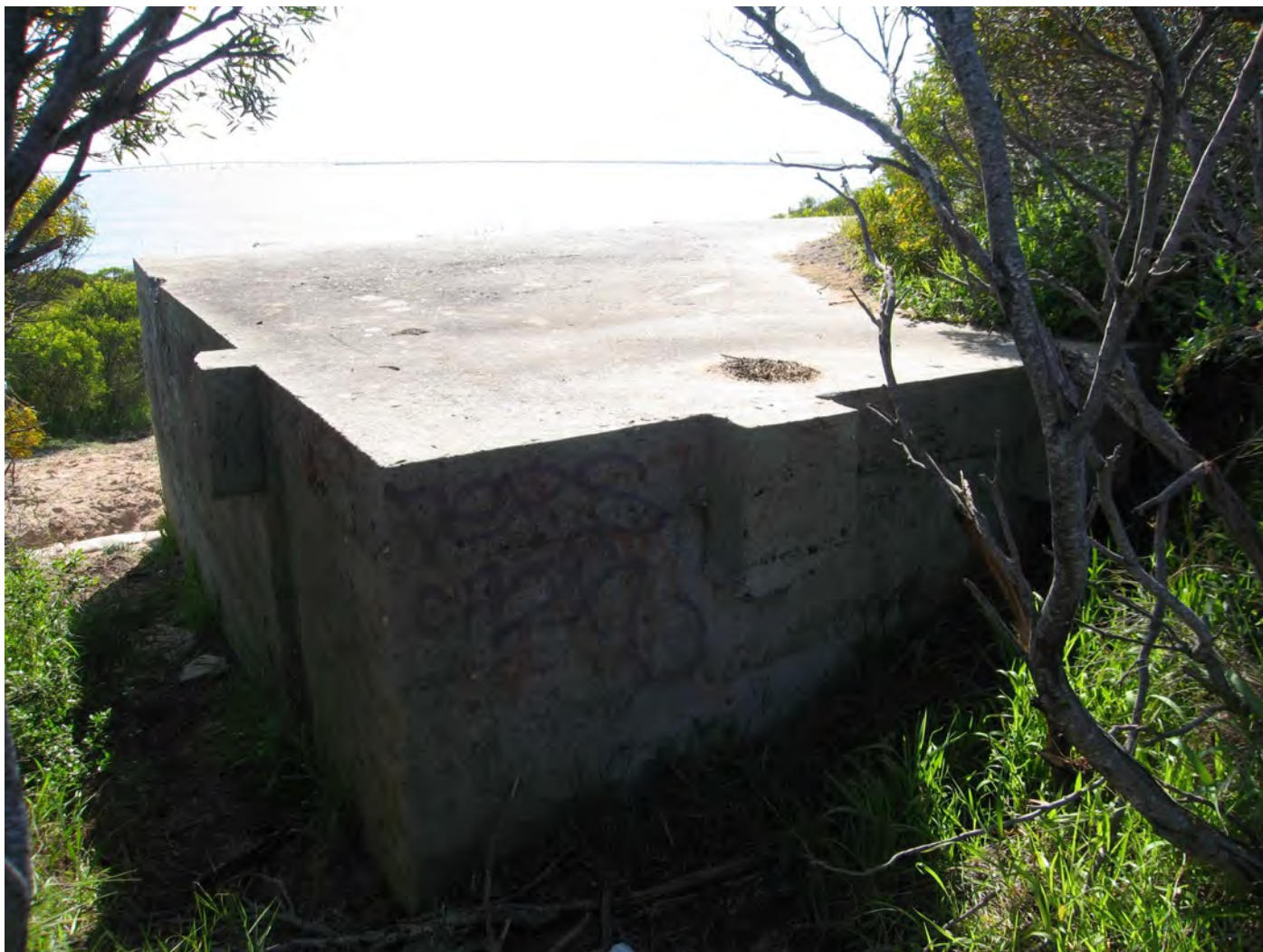
Figure 118: Ammunition Bunker – view across the roof
