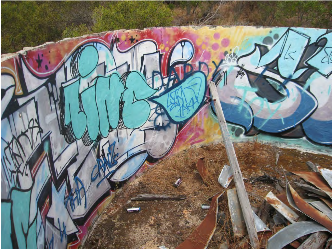
Figure 157: Water Tank interior
