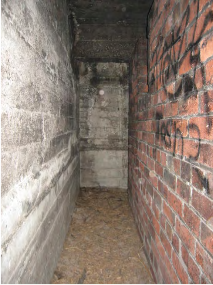
Figure 126: Ammunition Bunker – blast corridor between outer concrete wall and inner brick wall
