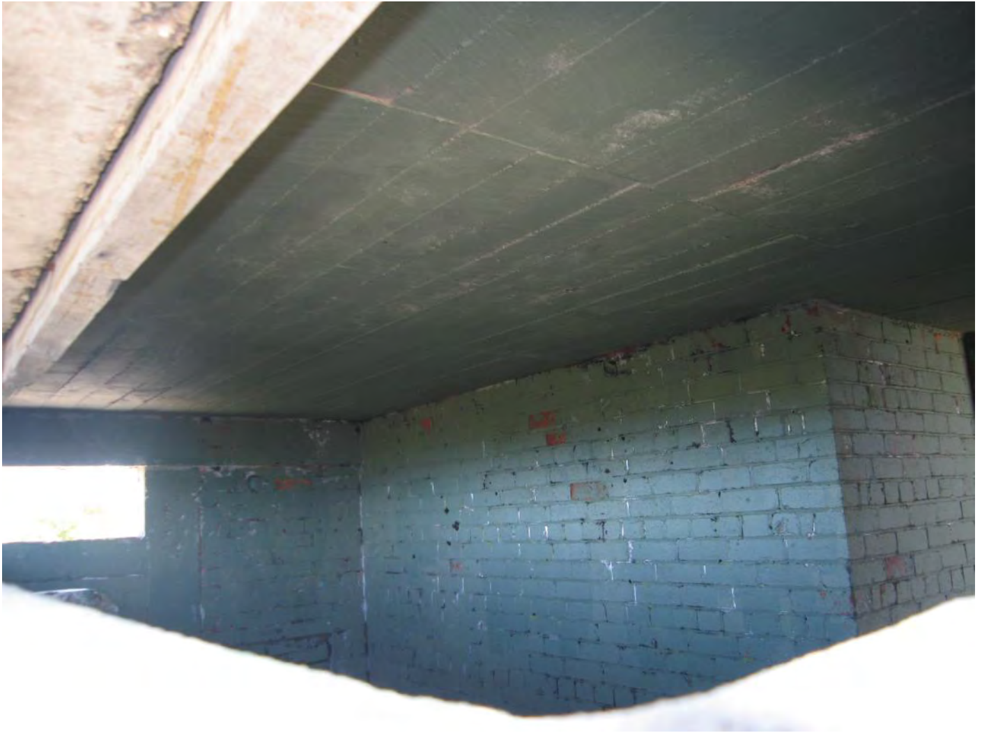
Figure 68: Concrete slab ceiling
