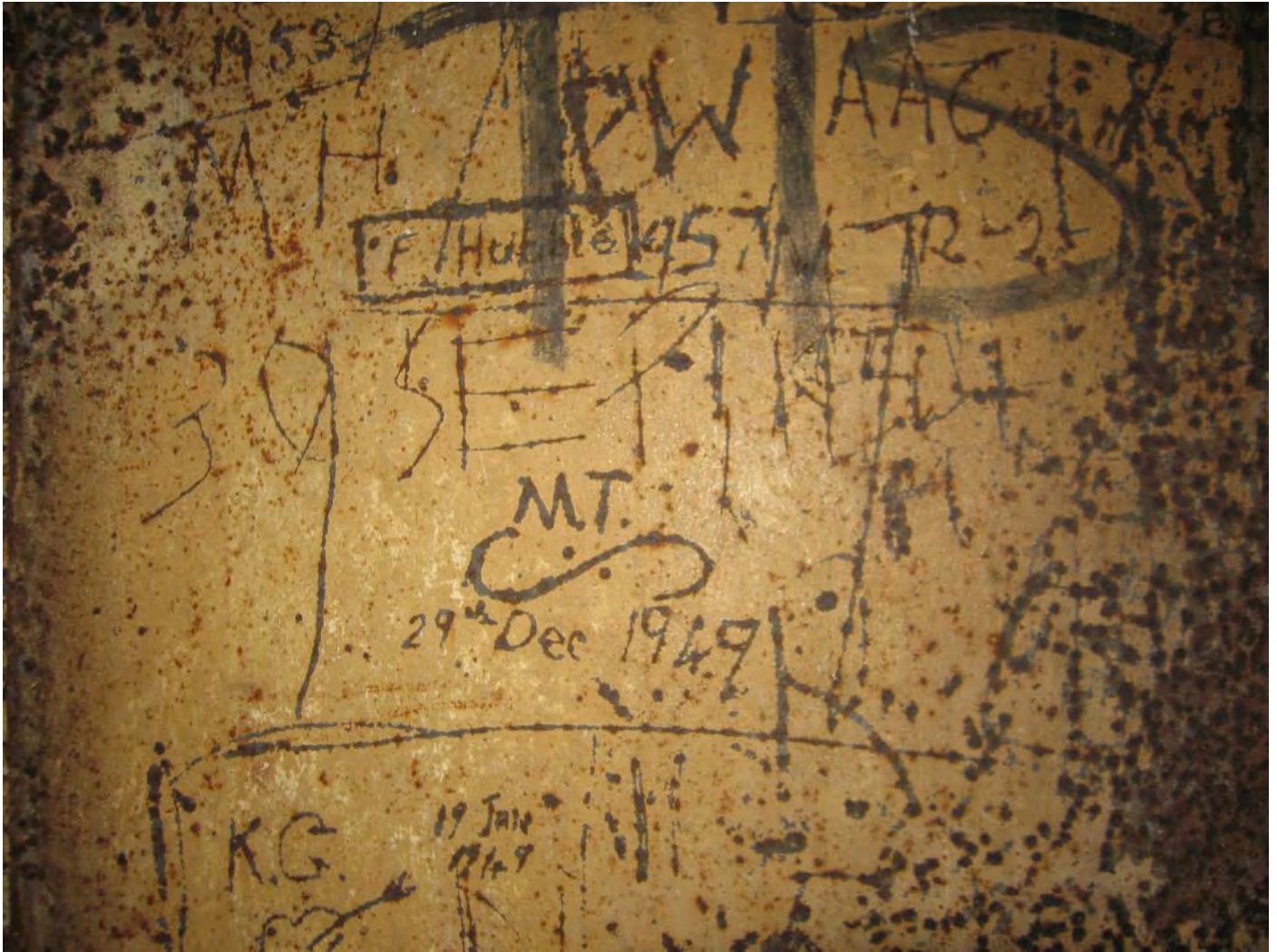
Figure 95: Operations Bunker – Graffiti scratched into entrance doors
