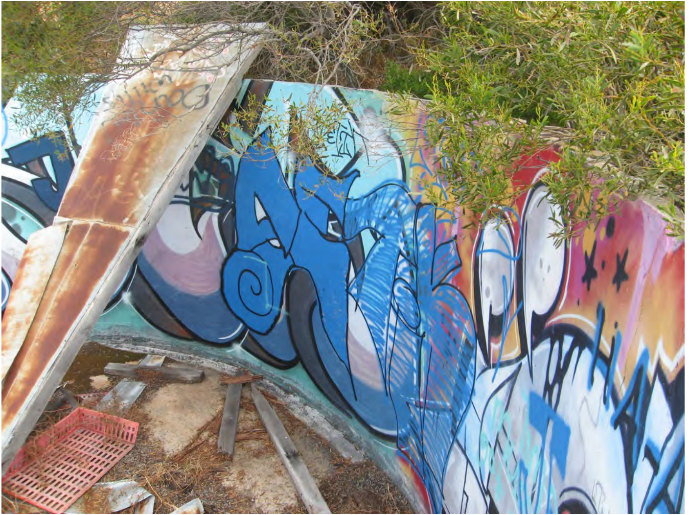
Figure 156: Water Tank Interior
