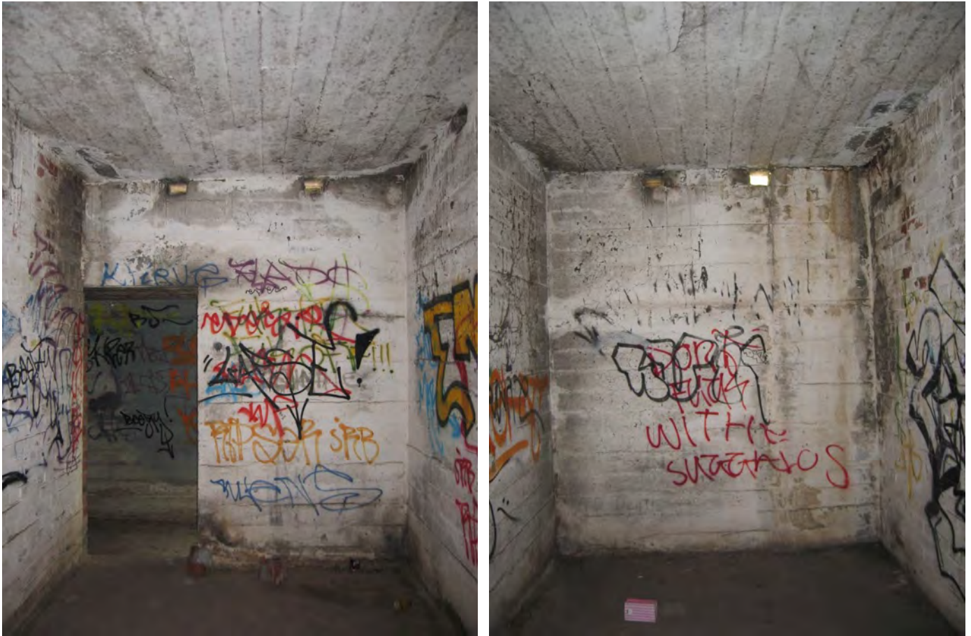
Figure 146: Ammunition Bunker - Room 1
