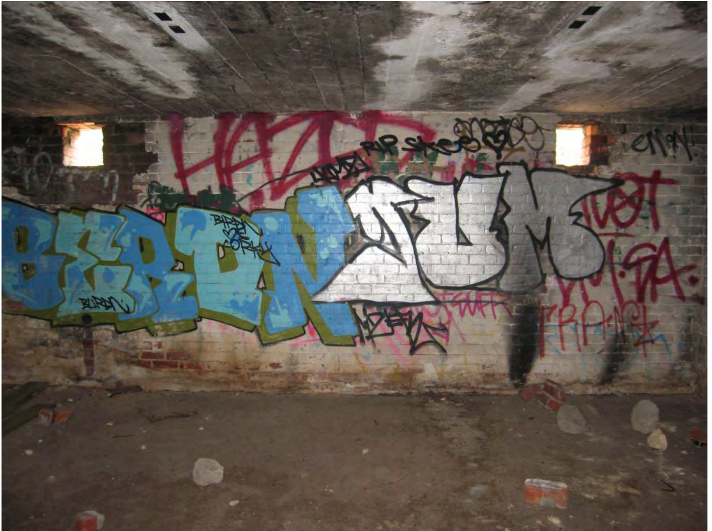
Figure 92: Operations Bunker – interior (north wall)
