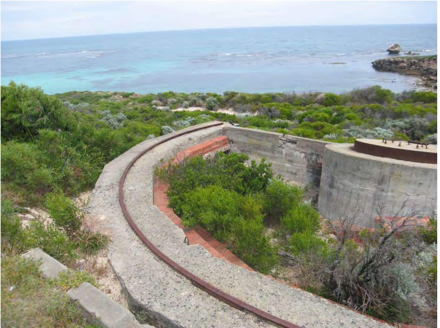
Figure 105: Gun Emplacement No. 1 – gun track
