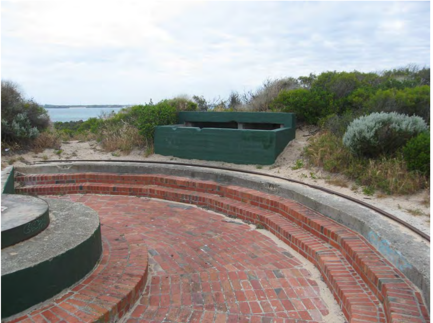
Figure 130: Gun Emplacement No. 2 – brick paving
