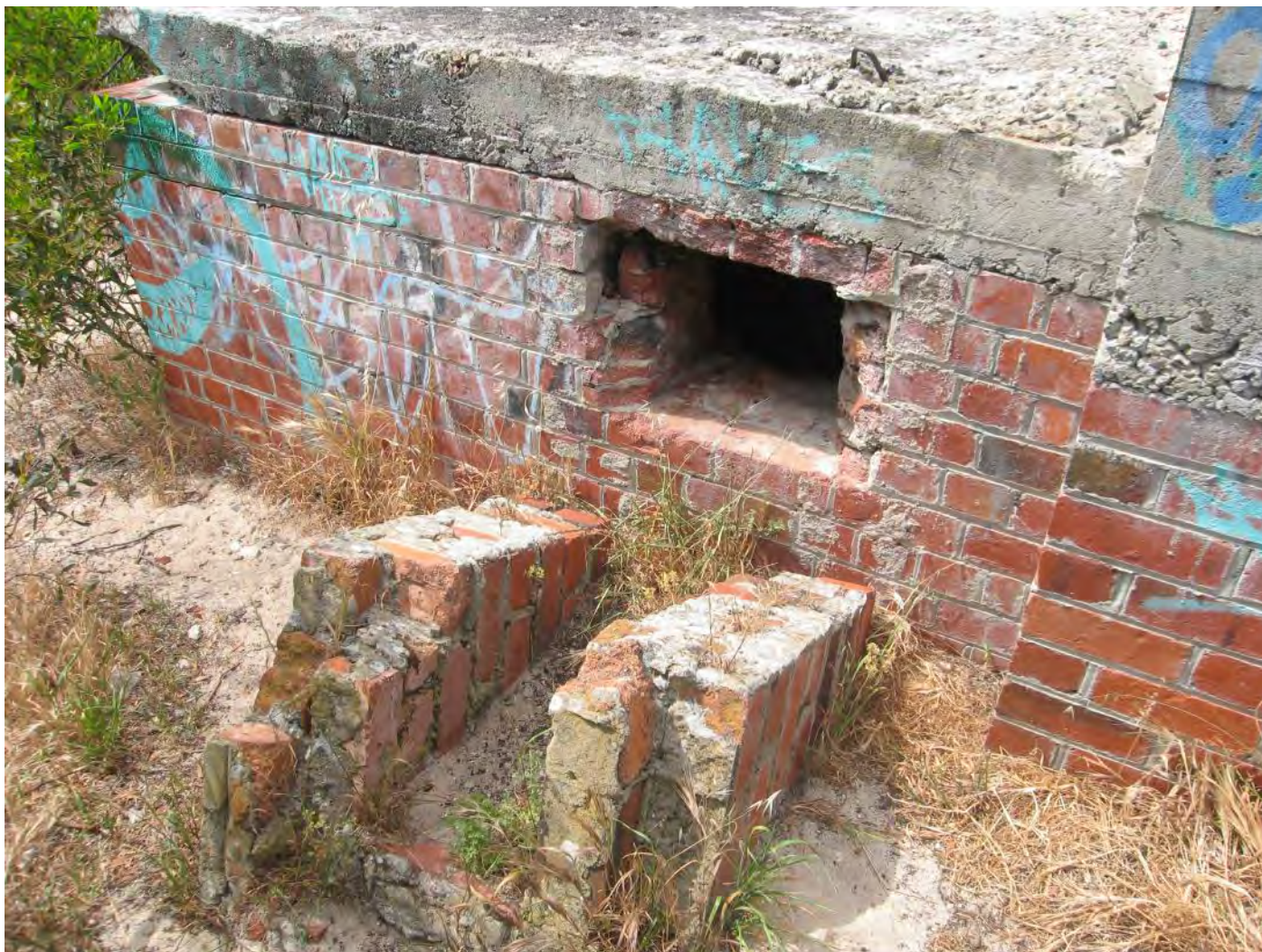
Figure 86: Operations Bunker – Openings in north elevation and remnant fabric
