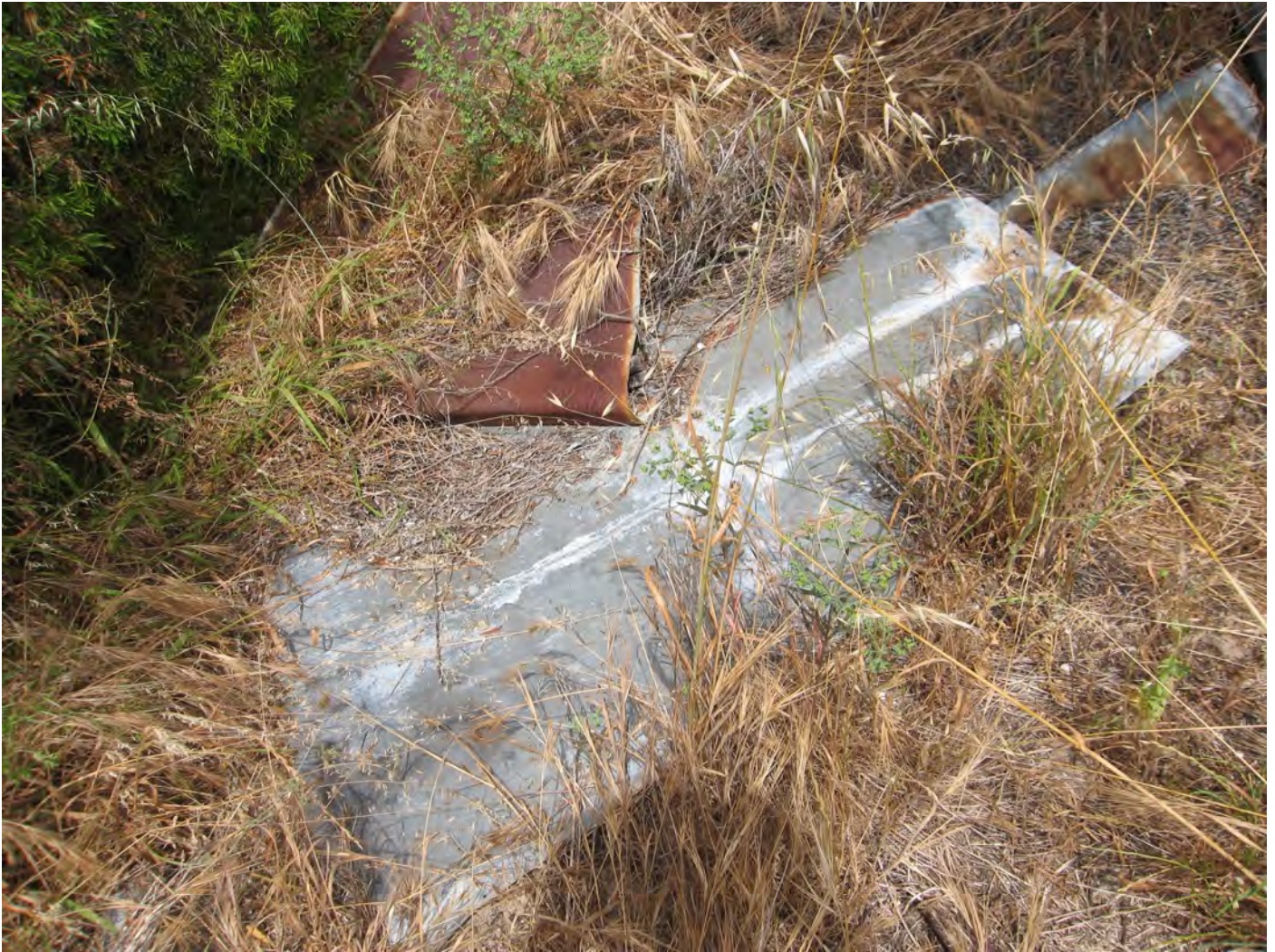
Figure 154: Water Tank – remnant roofing material
