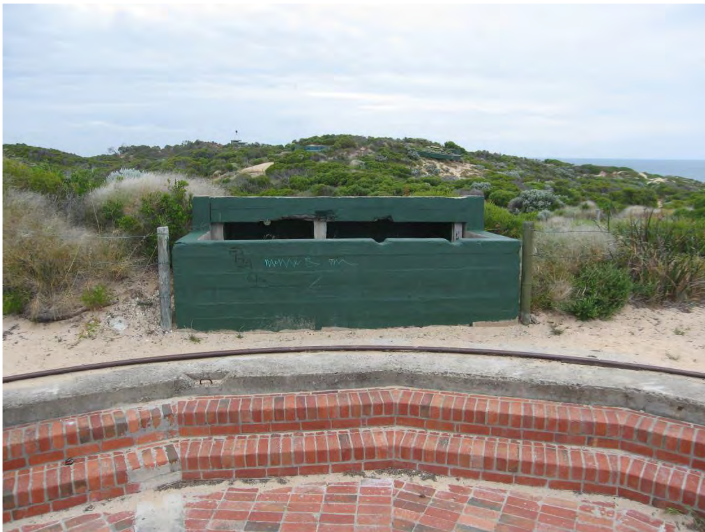
Figure 134: Gun Emplacement No. 2 – Ammunition Store 1
