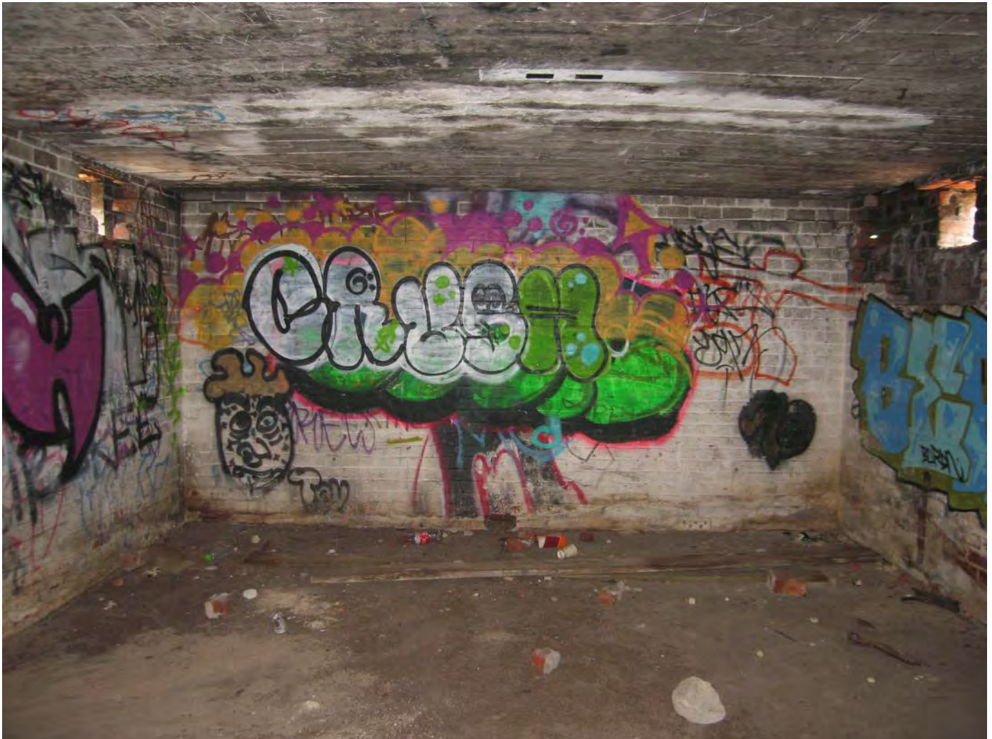
Figure 90: Operations Bunker – Interior (west wall)
