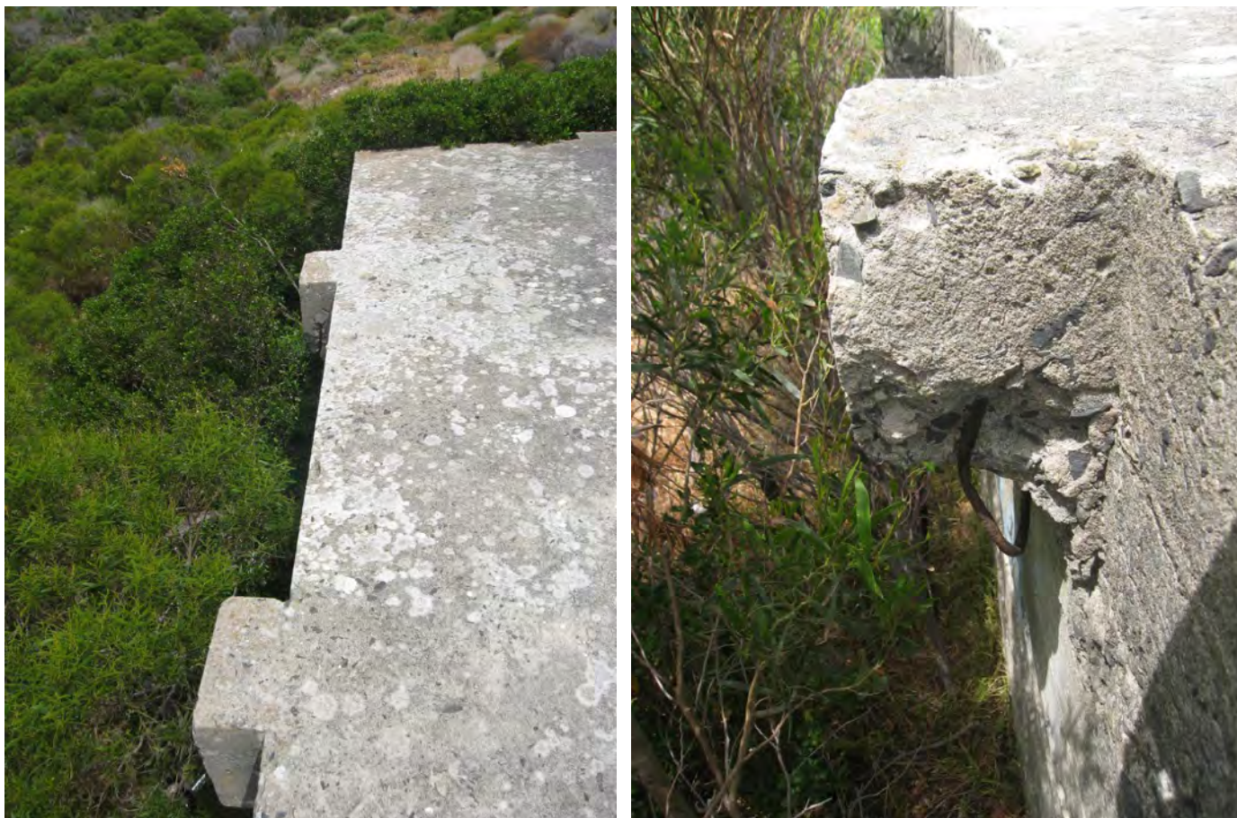
Figure 145: Ammunition Bunker No. 2 – Ventilation shafts
