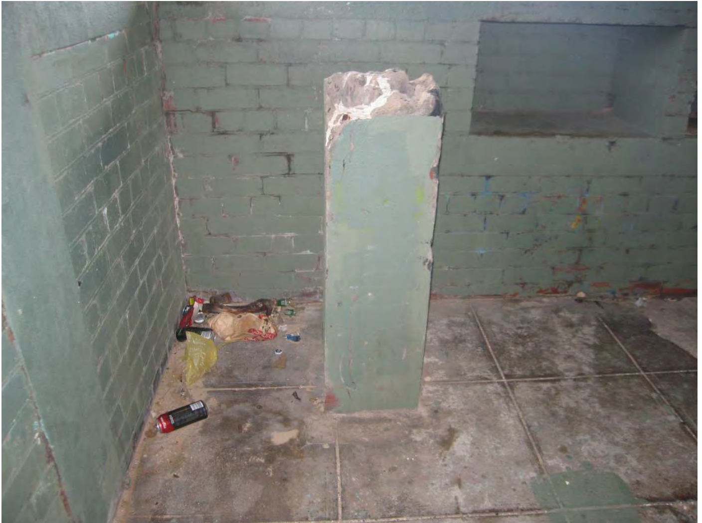
Figure 71: Reinforced concrete observation mounts
