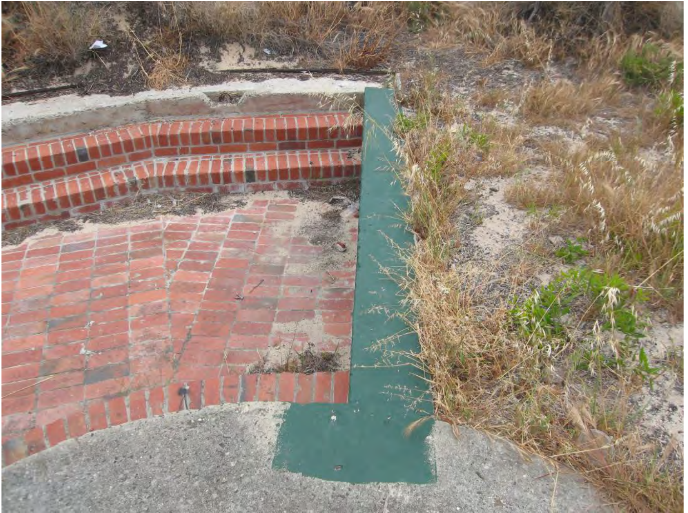
Figure 132: Gun Emplacement No. 2 – terminating concrete wall
