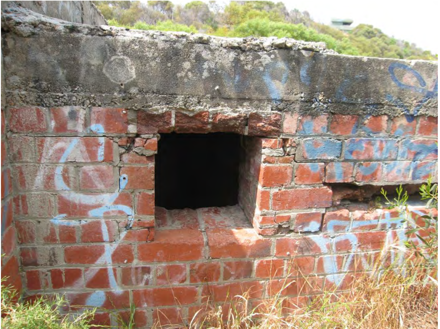
Figure 85: Operations Bunker – Openings in north wall
