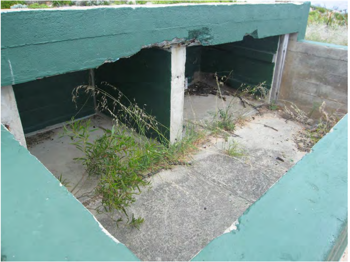
Figure 136: Gun Emplacement No. 2 – Ammunition Store 1
