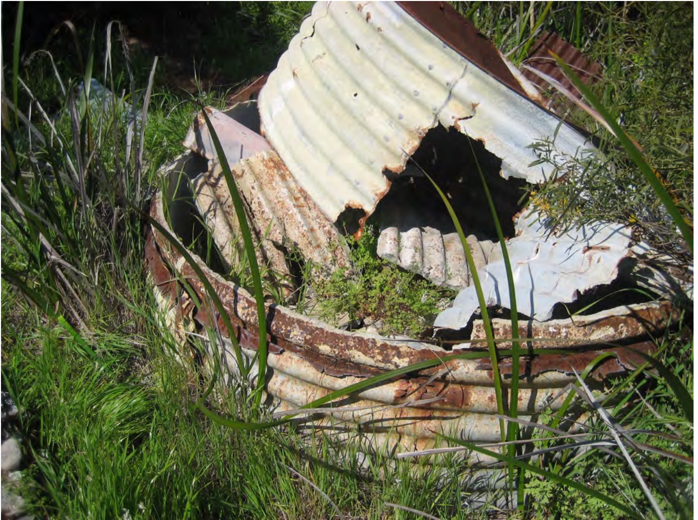
Figure 161: Former Well cladding
