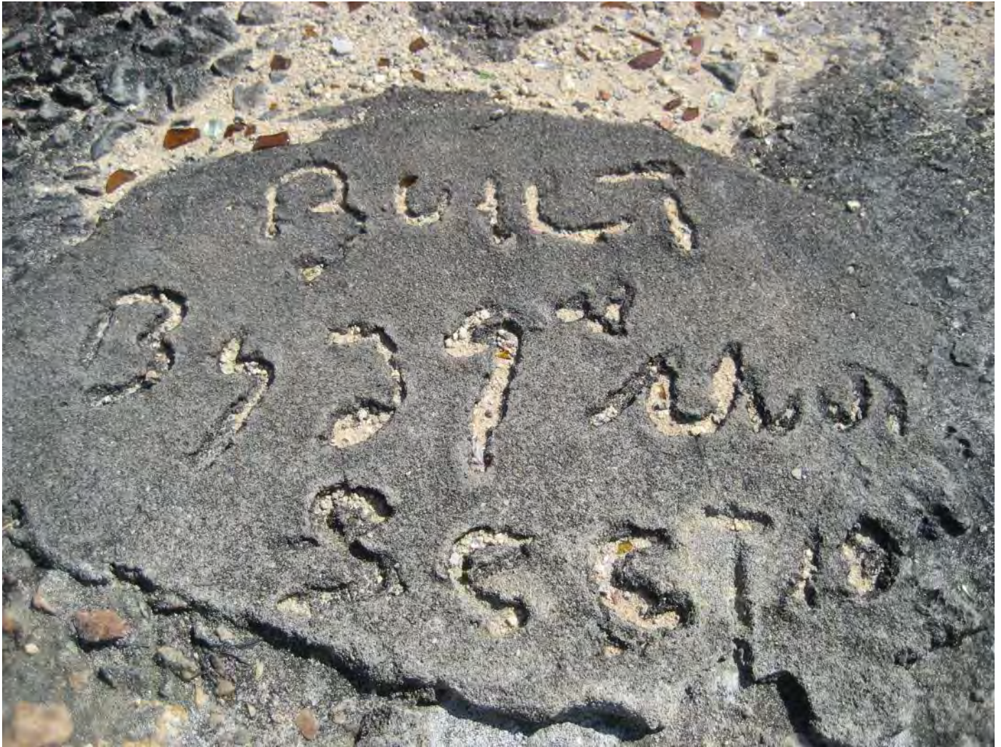
Figure 83: Operations Bunker – Roof inscription
