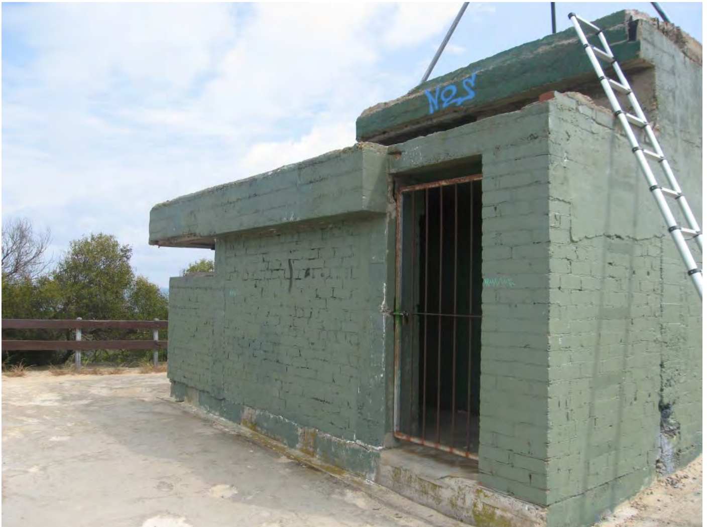
Figure 56: Observation Post – South Elevation
