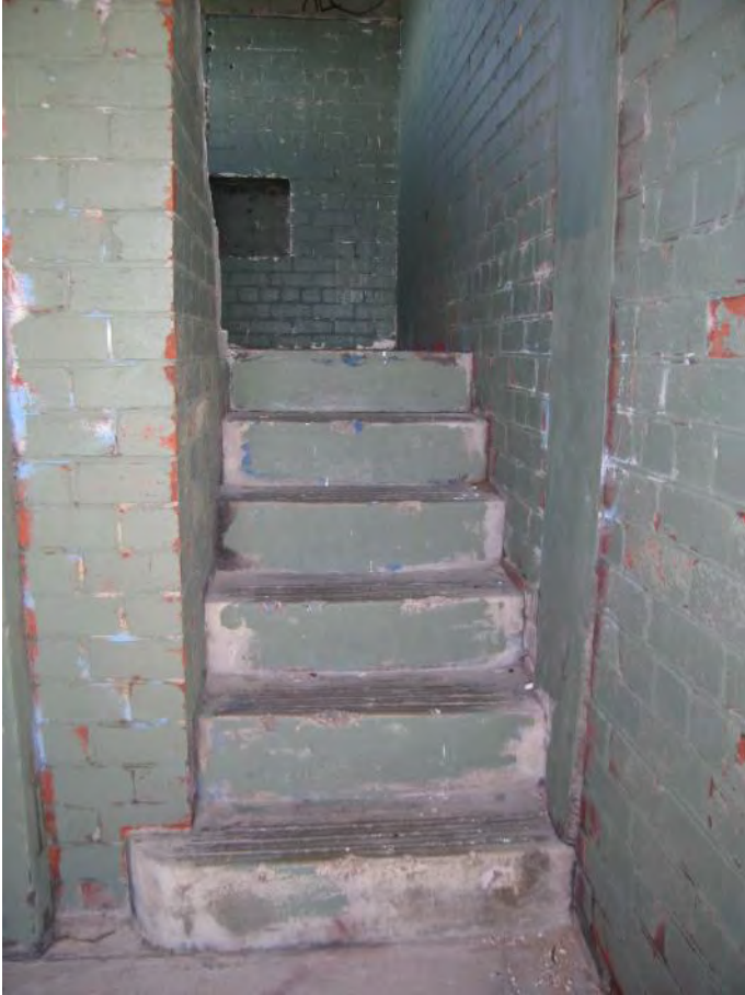
Figure 69: Stairs to upper level
