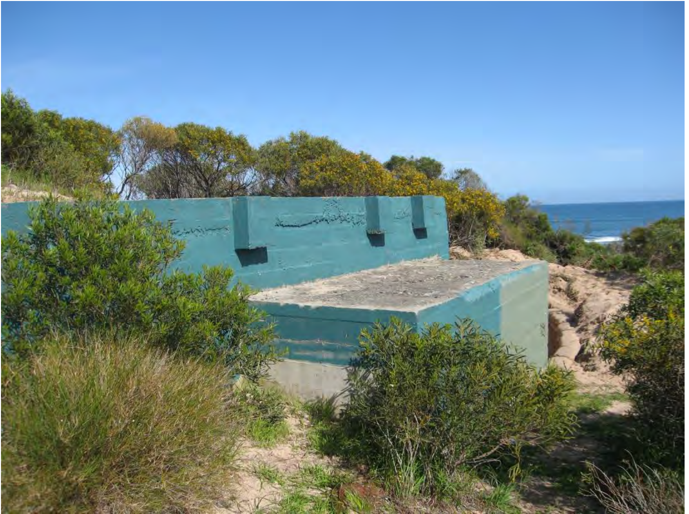
Figure 117: Ammunition Bunker – East elevation
