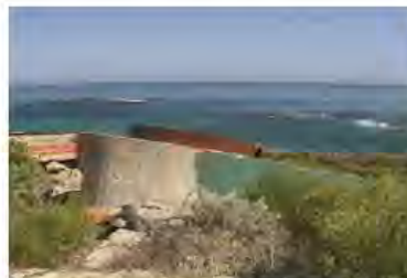
PHOTO: The coastal defence battery at Point Peron has fallen into disrepair. (ABC News)
