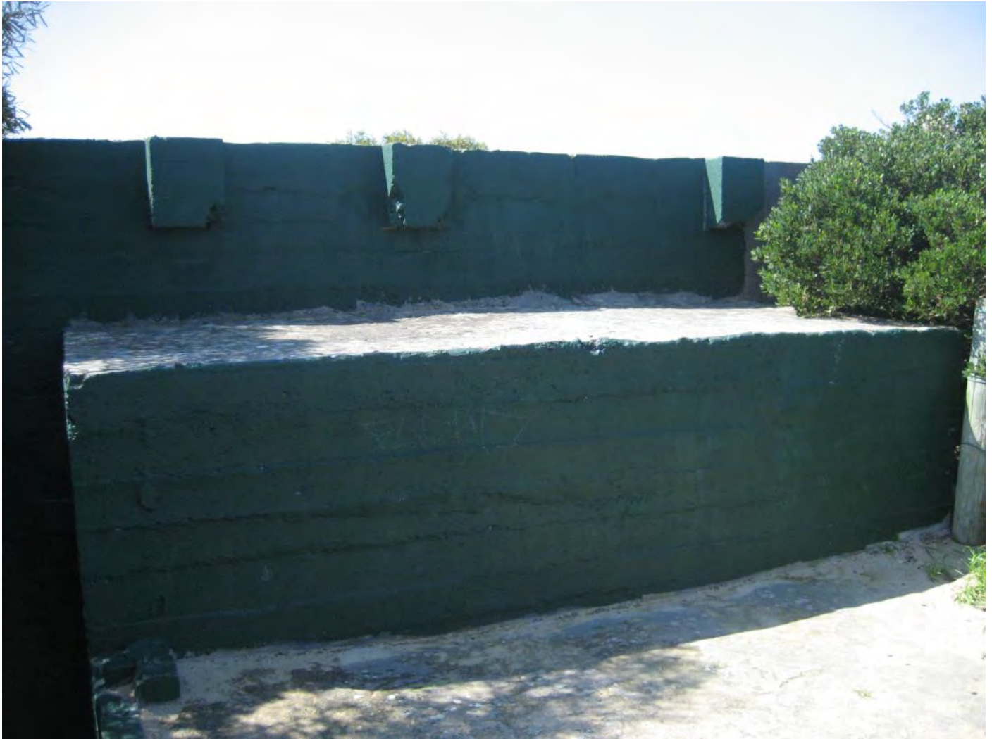
Figure 142: Ammunition Bunker No. 2 – south-west elevation
