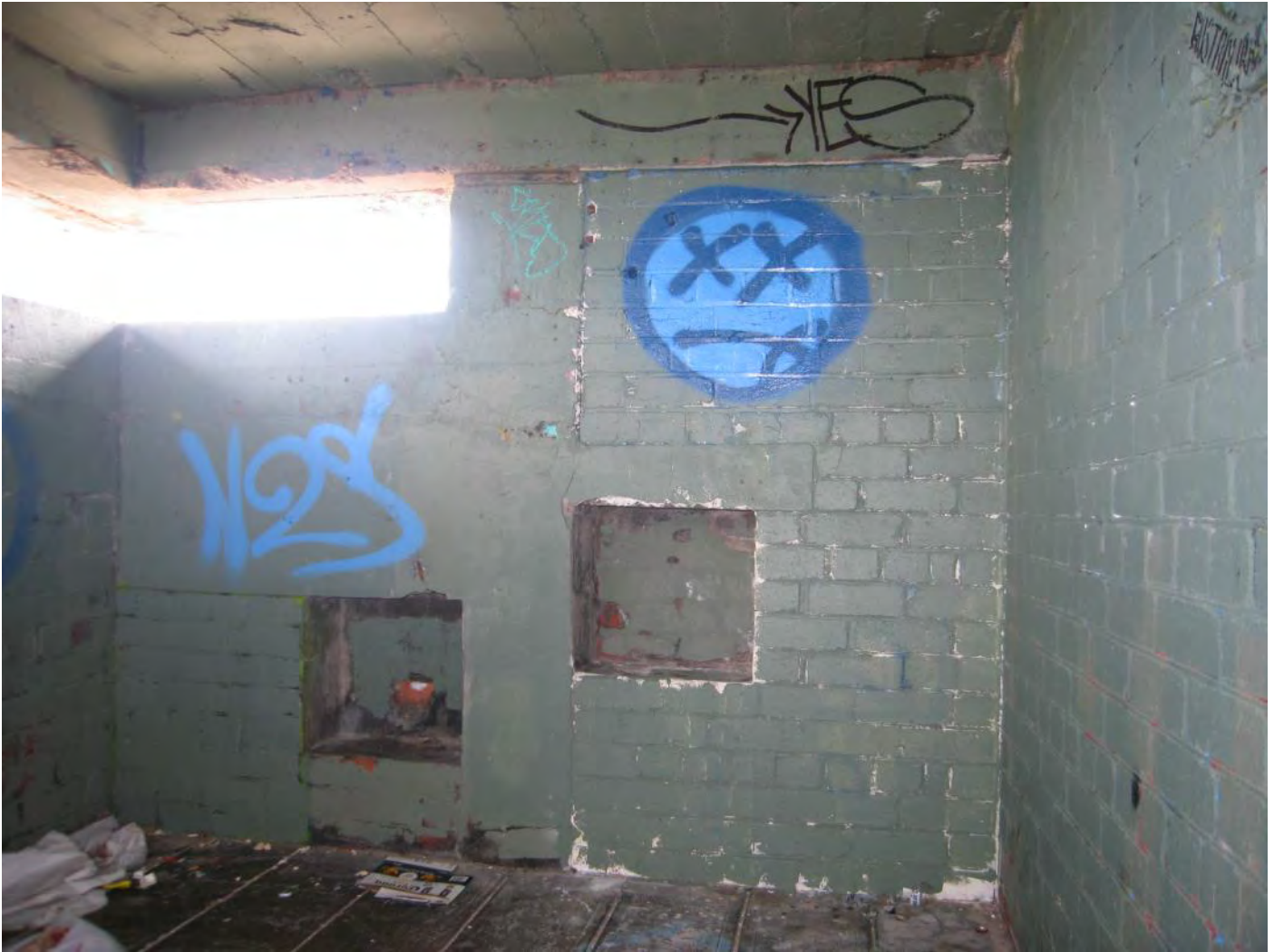
Figure 73: Storage areas incorporated into the north wall of the upper level
