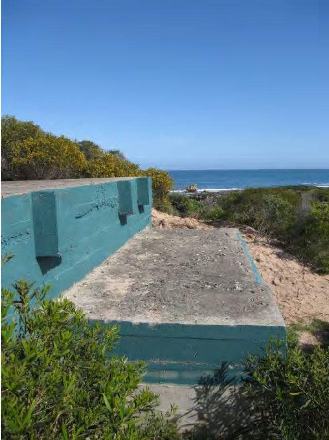
Figure 119: Ammunition Bunker – roof to entry tunnel
