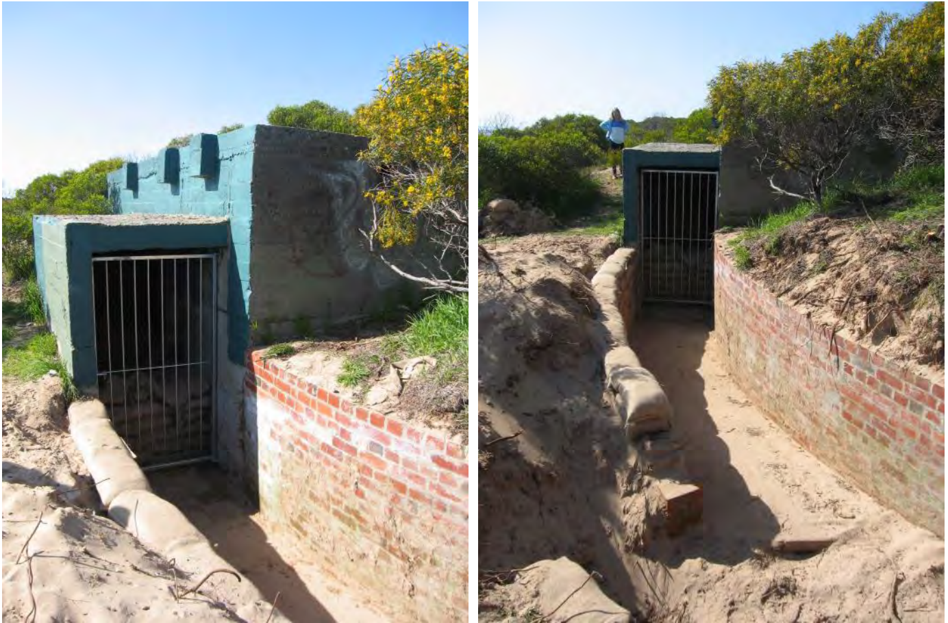
Figure 116: Ammunition Bunker - entrance
