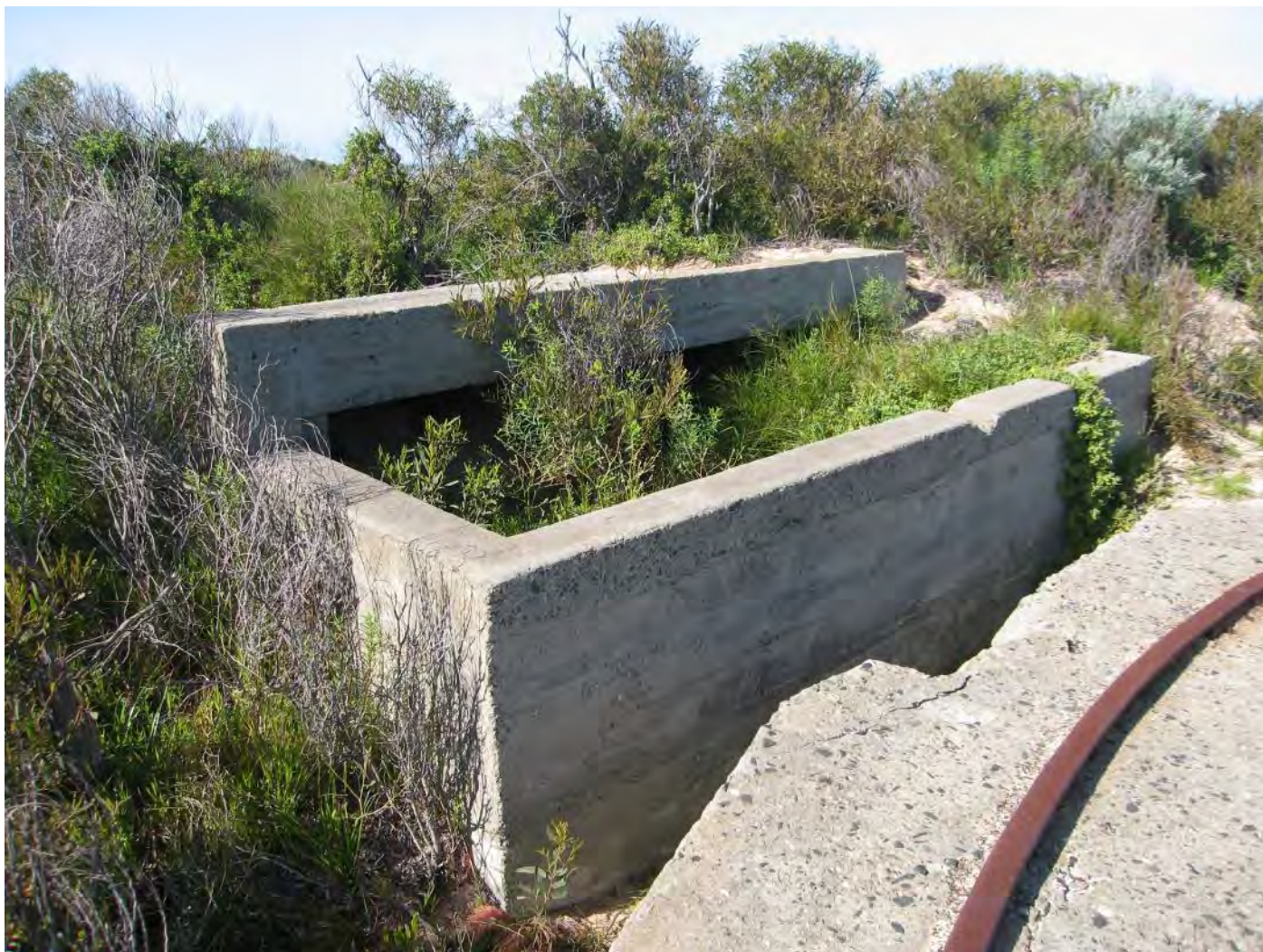
Figure 111: Gun Emplacement - Ammunition Store No. 2
