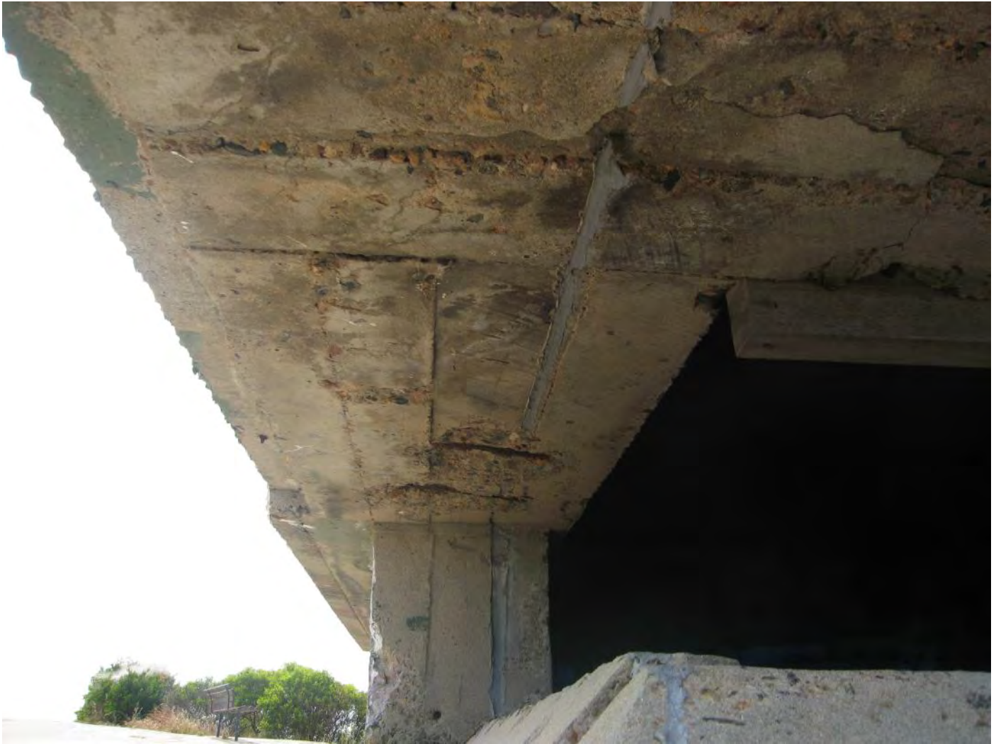
Figure 61: Underside of Concrete Overhang to Observation Opening
