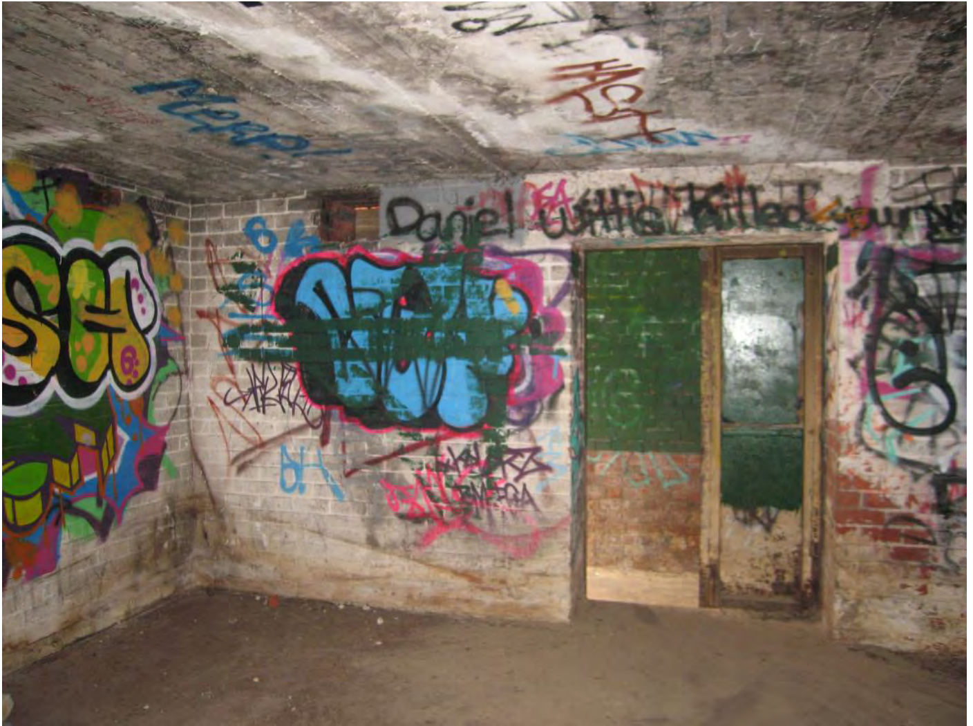
Figure 91: Operations Bunker – Interior (south wall)
