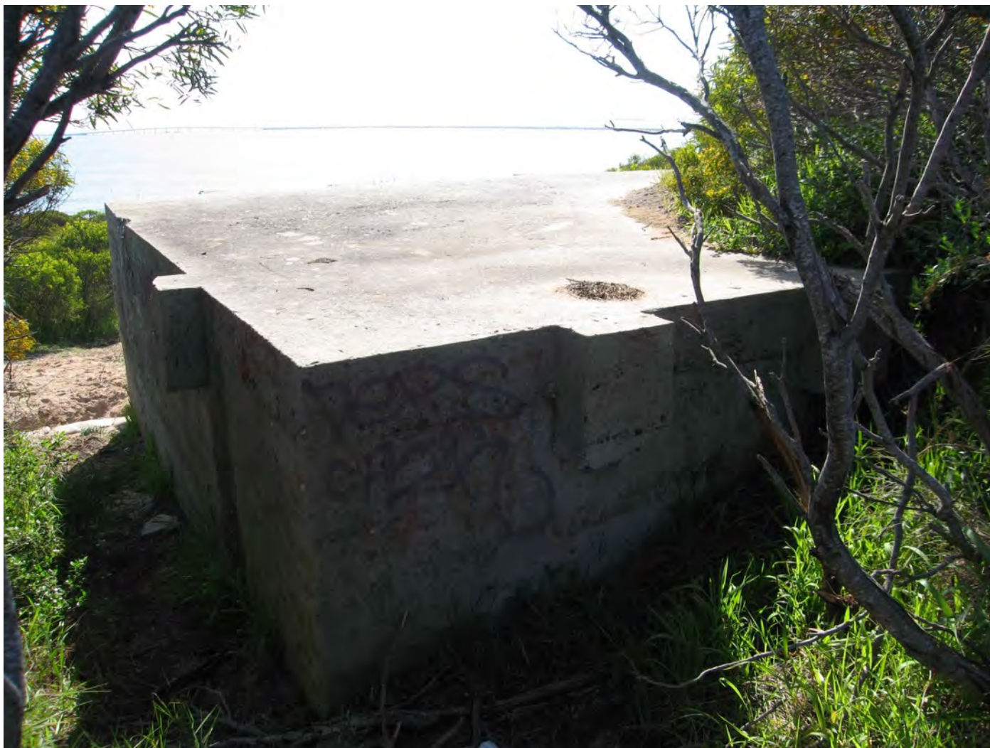
Figure 118: Ammunition Bunker – view across the roof
