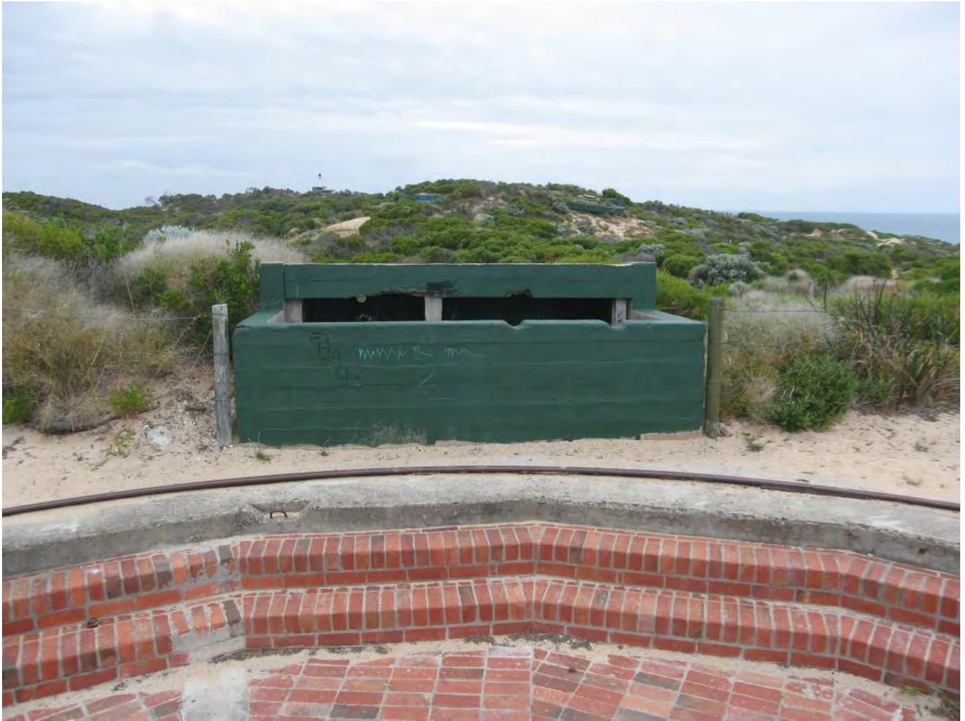
Figure 134: Gun Emplacement No. 2 – Ammunition Store 1
