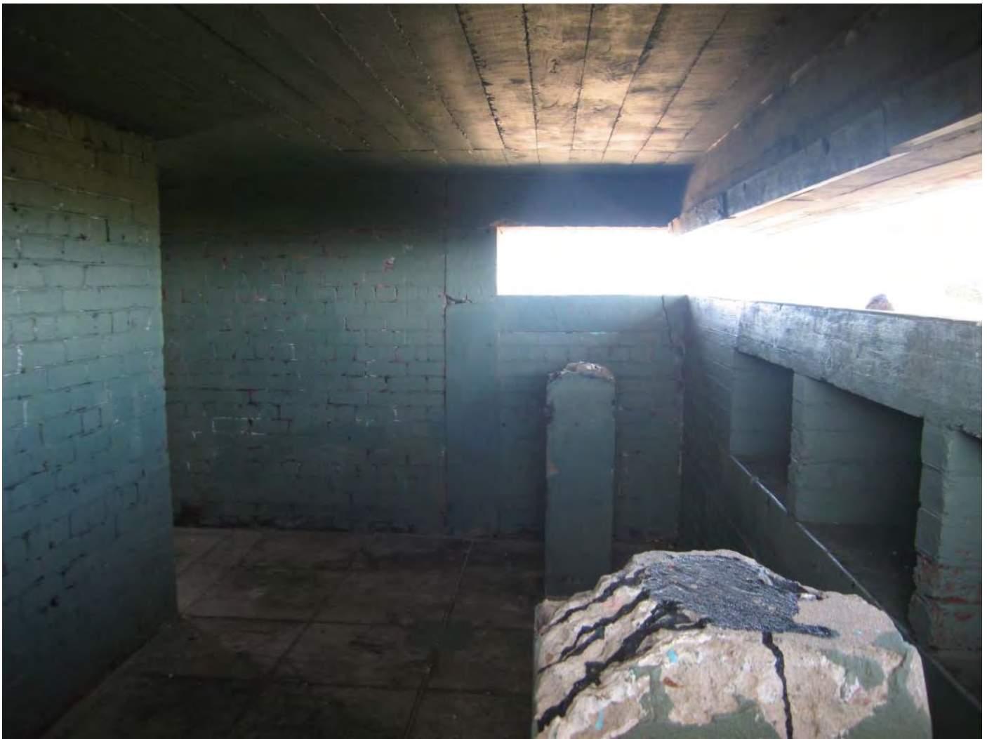
Figure 67: Ground level interior
