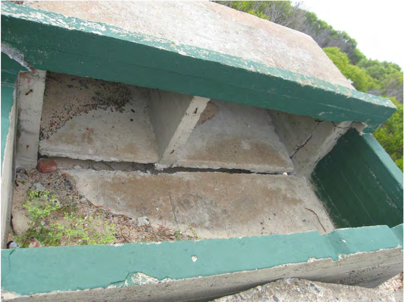
Figure 107: Gun Emplacement - Ammunition Store No. 1
