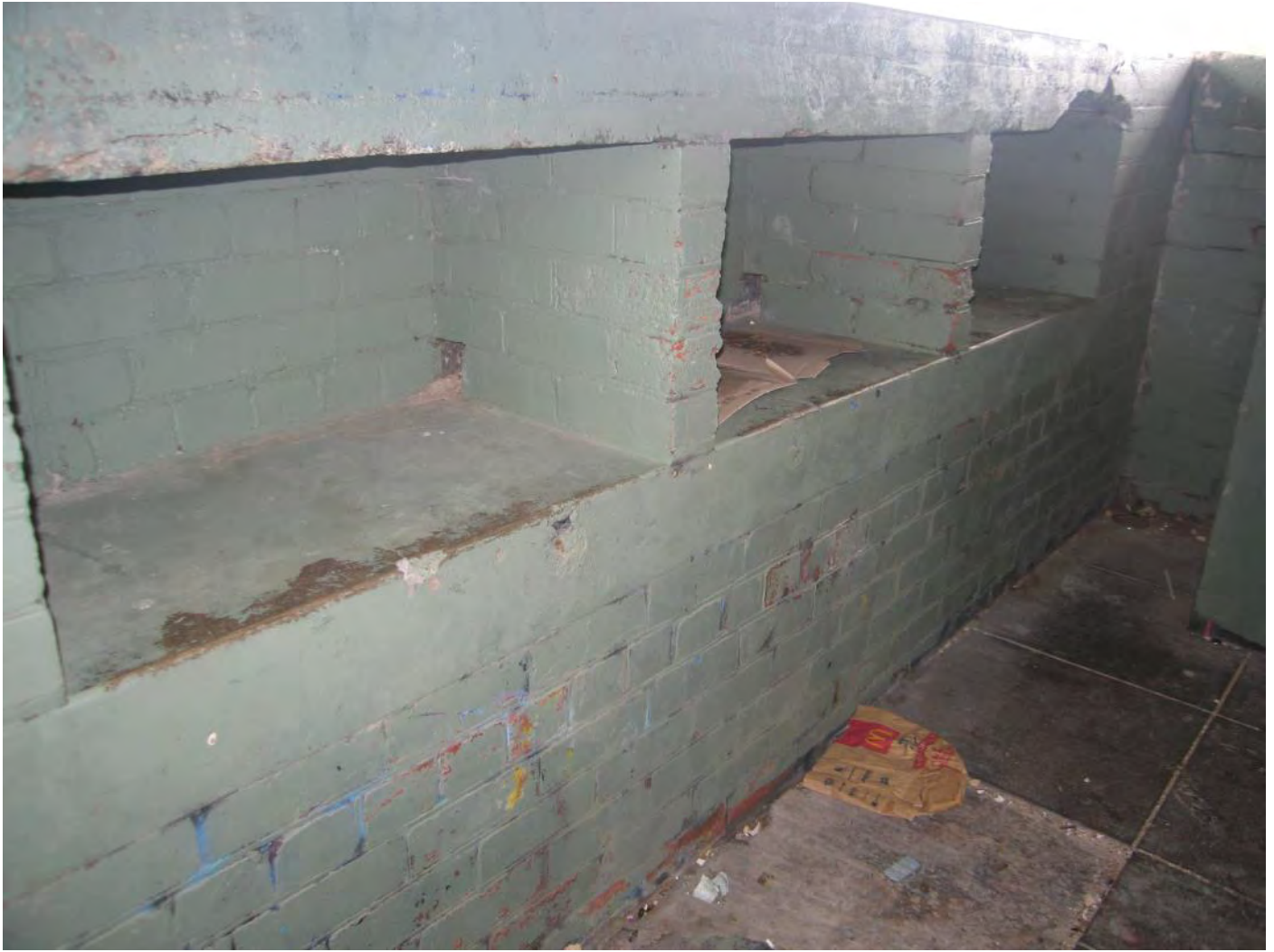
Figure 72: Storage incorporated into the west wall
