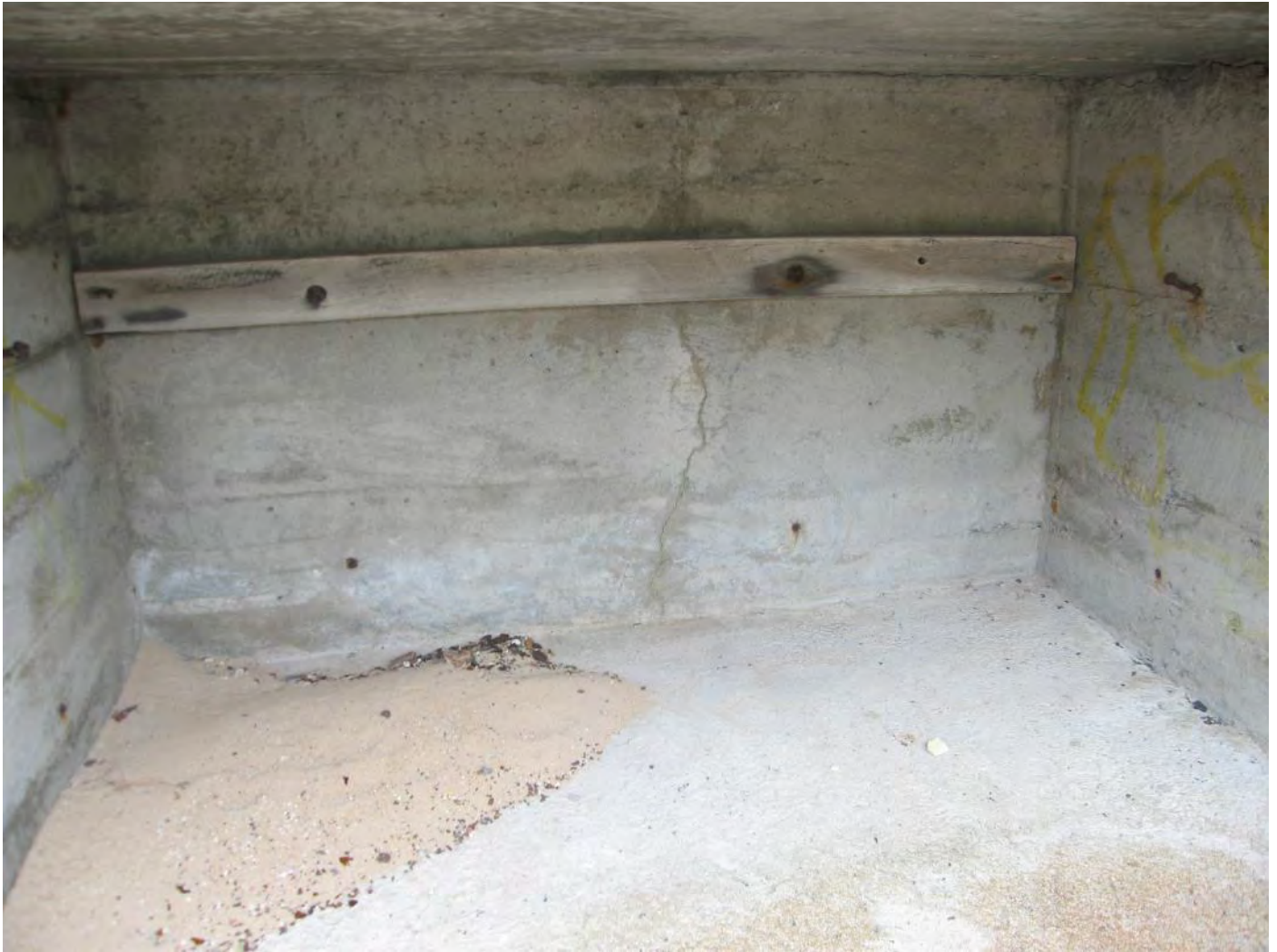
Figure 109: Gun Emplacement - Ammunition Store No. 1
