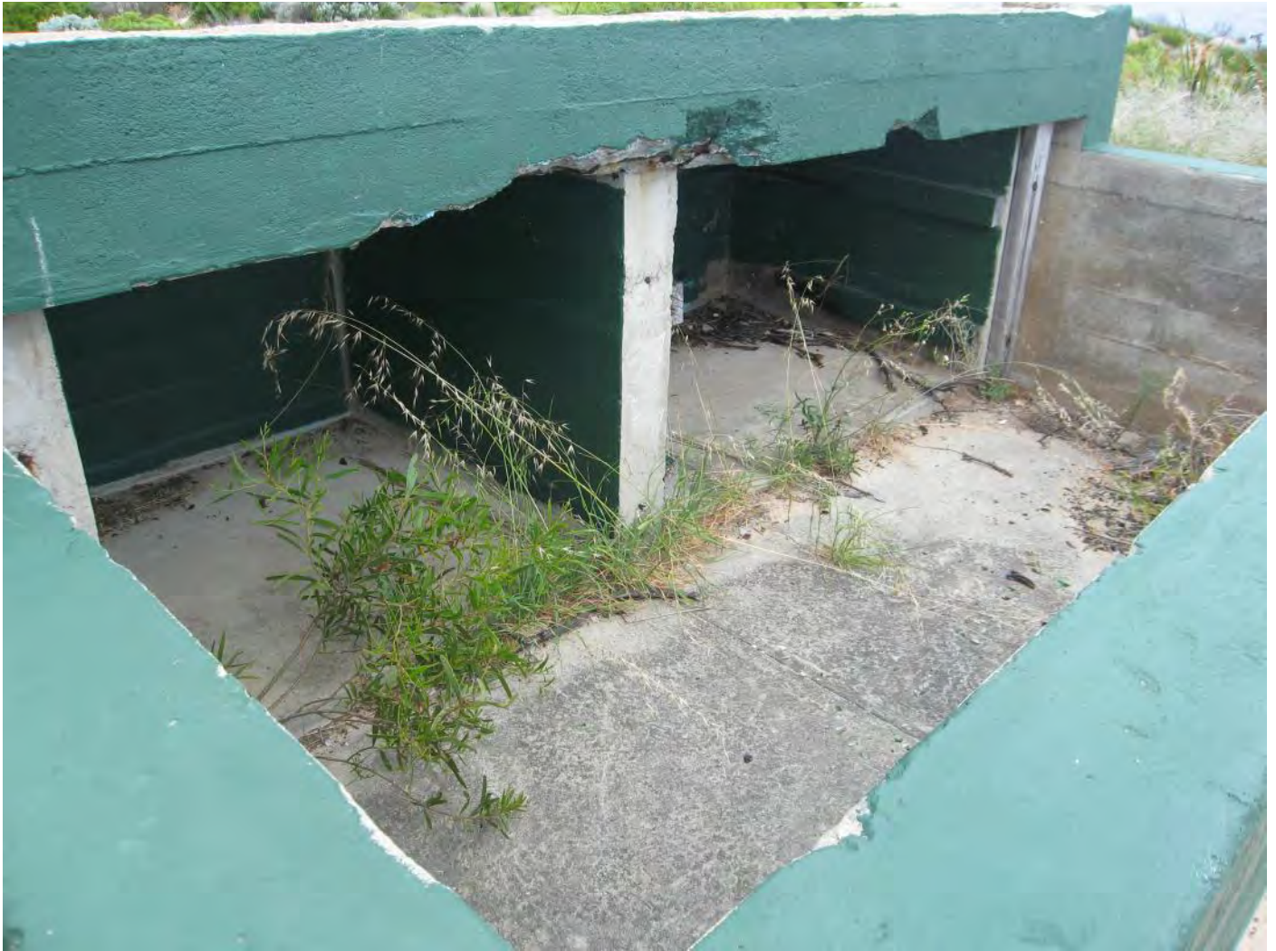
Figure 136: Gun Emplacement No. 2 – Ammunition Store 1
