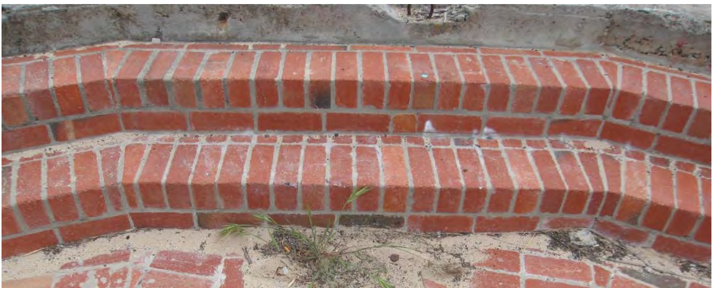
Figure 131: Gun Emplacement No. 2 – brick steps
