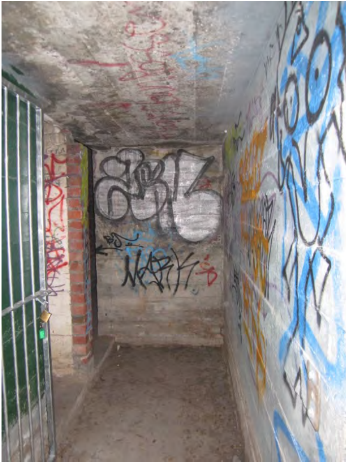
Figure 147: Entry tunnel leading to the two internal rooms
