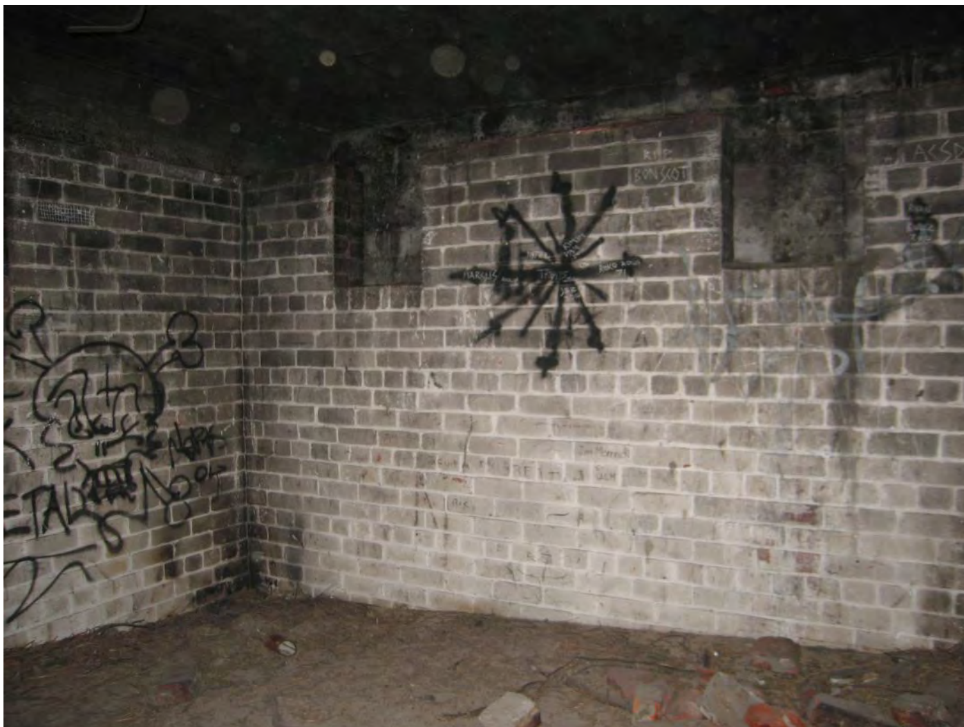
Figure 124: Ammunition Bunker – Room 2
