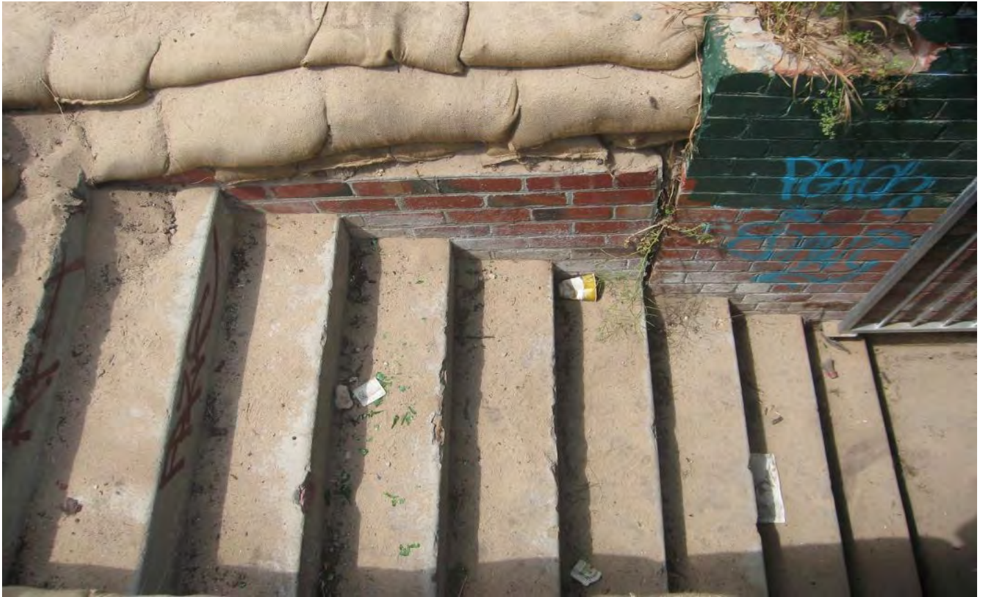
Figure 88: Operations Bunker – Steps down to the entrance
