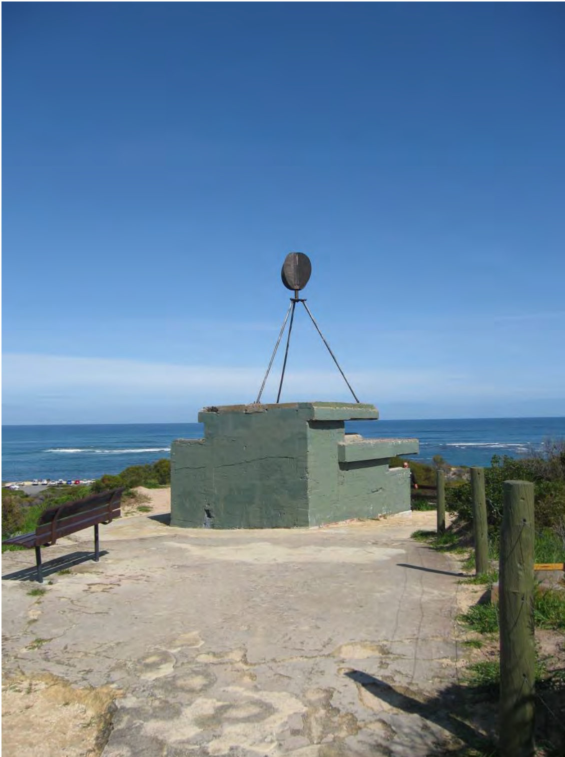
Figure 53: Observation Post - East and North Elevations
