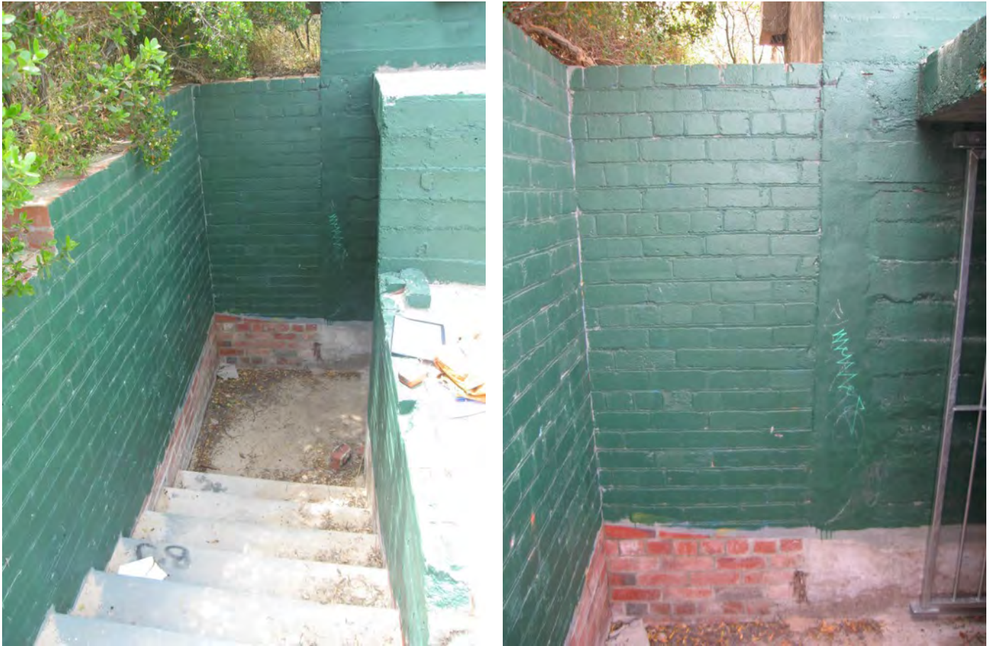
Figure 143: Ammunition Bunker No. 2 – Entrance
