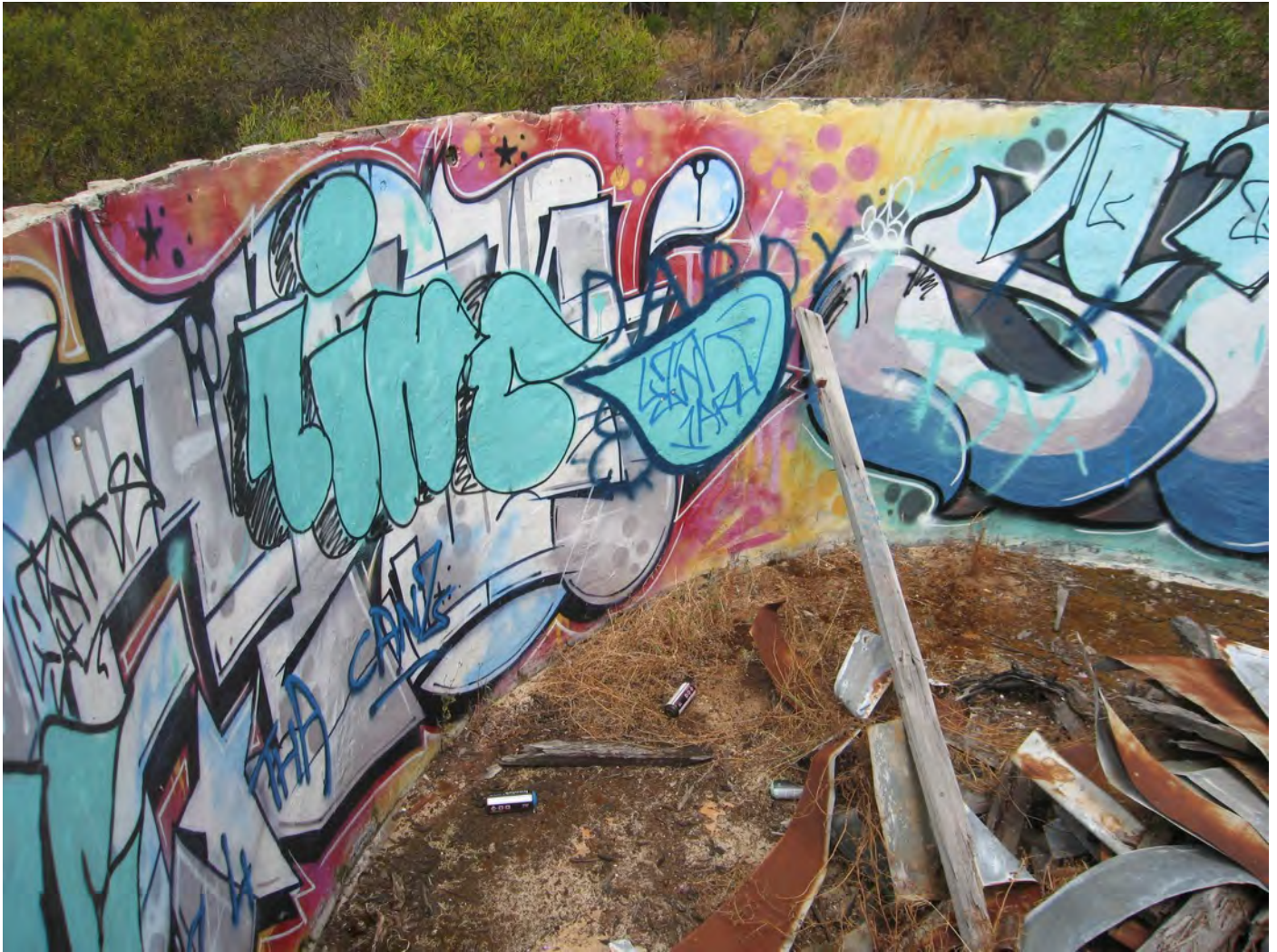
Figure 157: Water Tank interior
