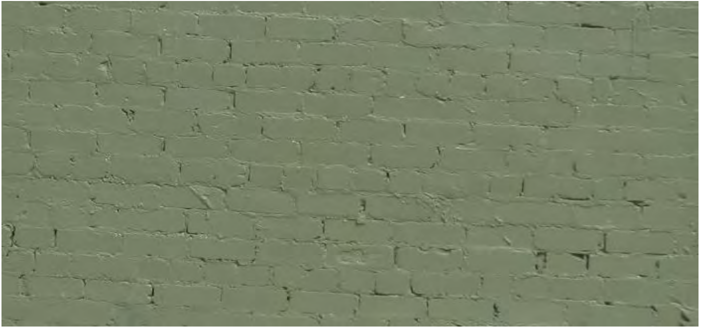
Figure 55: English Garden Bond Brickwork
