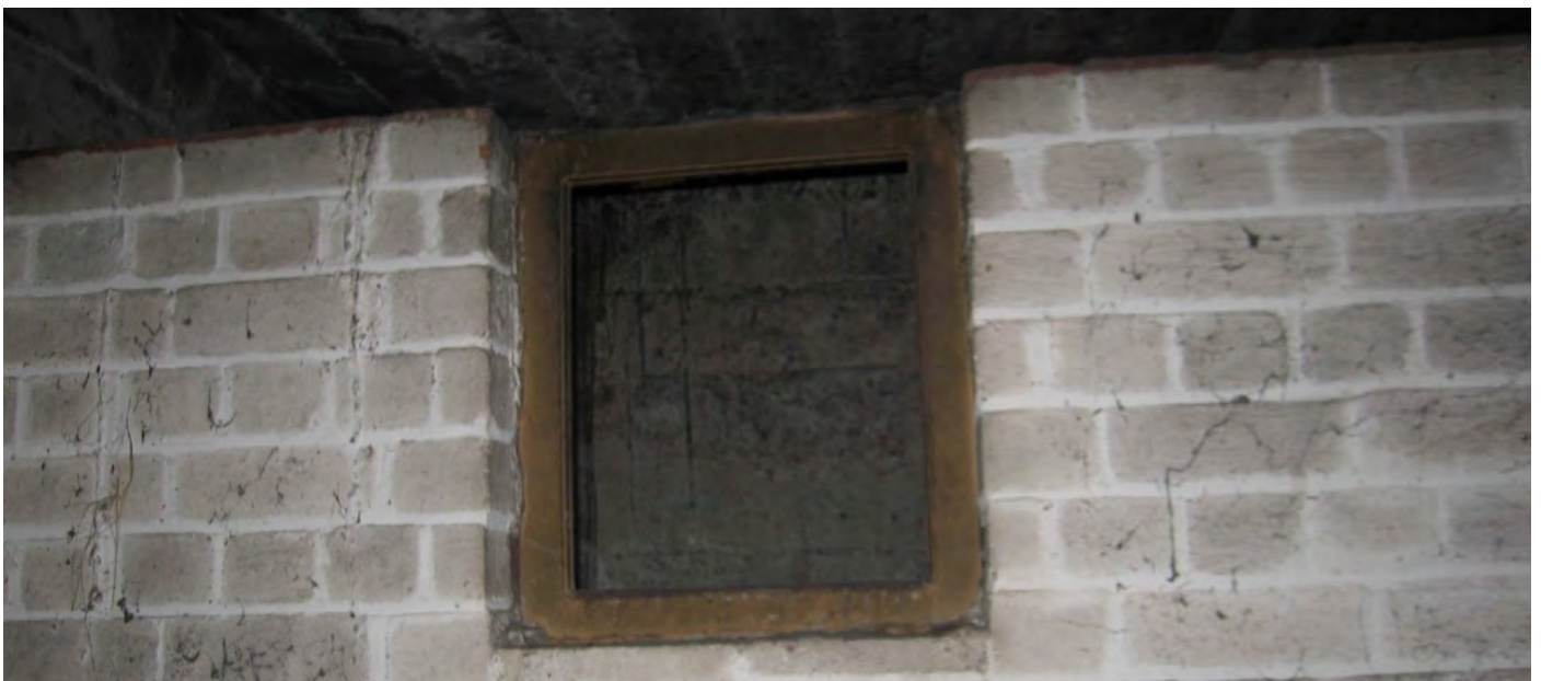
Figure 148: Ventilation openings in Room 2
