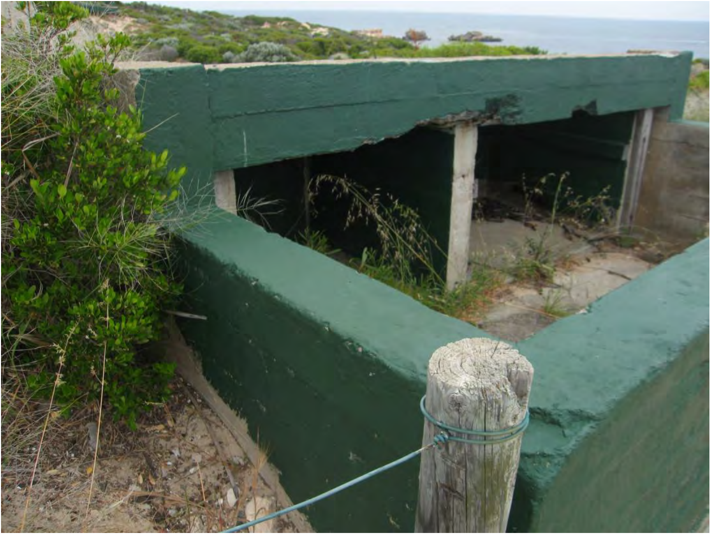
Figure 135: Gun Emplacement No. 2 – Ammunition Store 1
