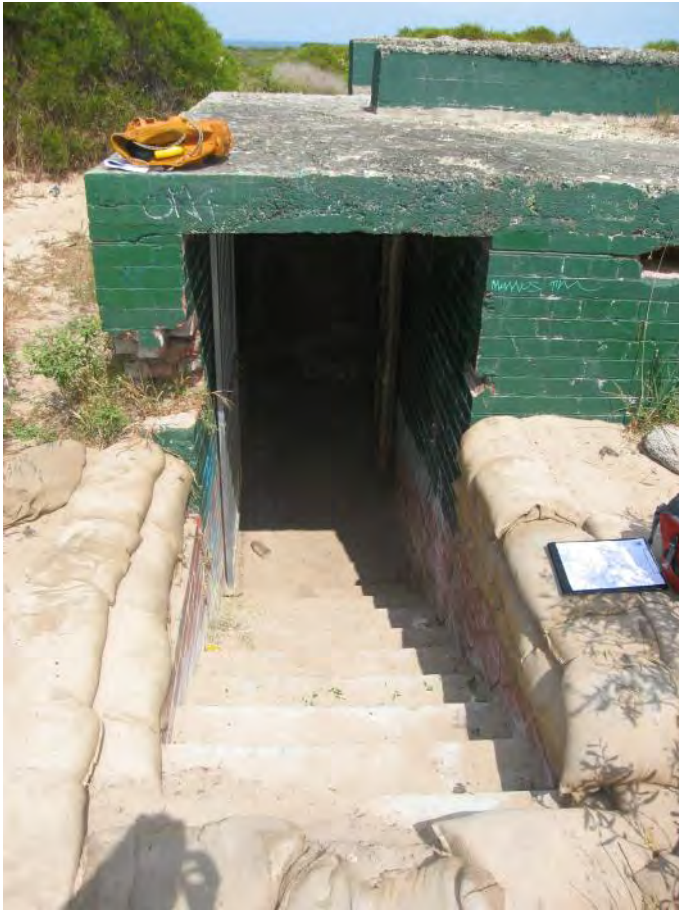
Figure 78: Operations Bunker – steps down to the entrance
