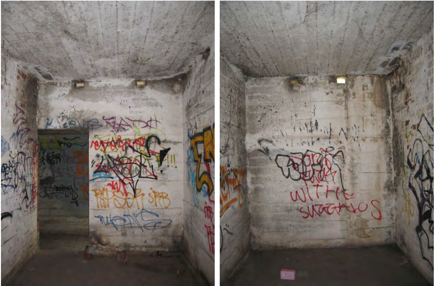
Figure 146: Ammunition Bunker - Room 1
