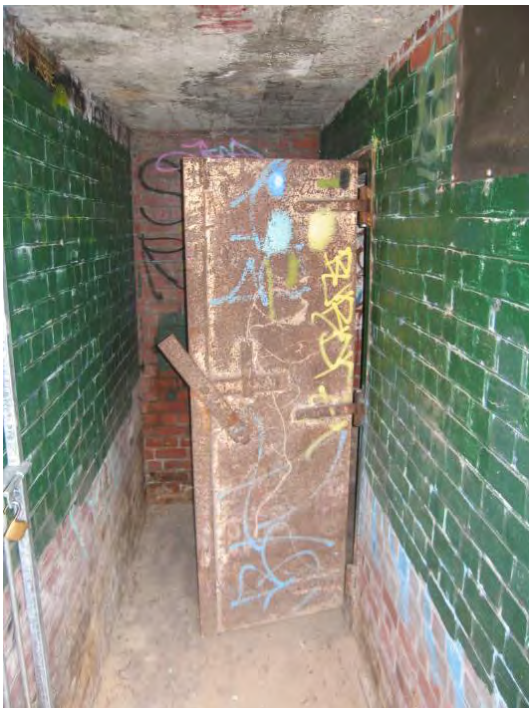
Figure 89: Operations Bunker – Extant steel entrance doors
