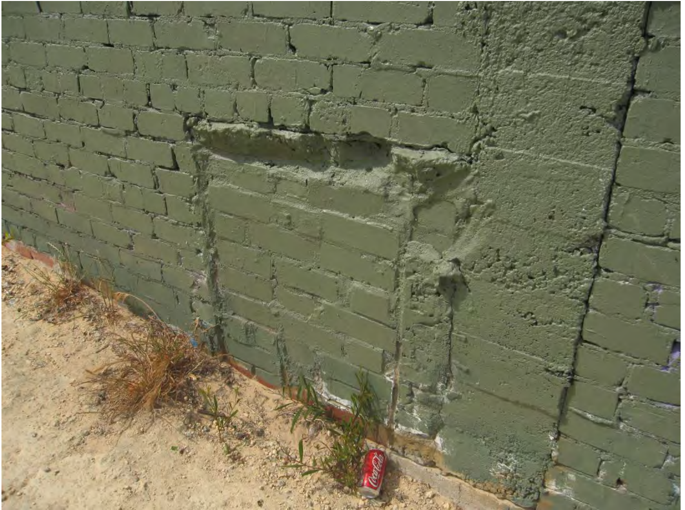
Figure 64: North Elevation – brick infill panel
