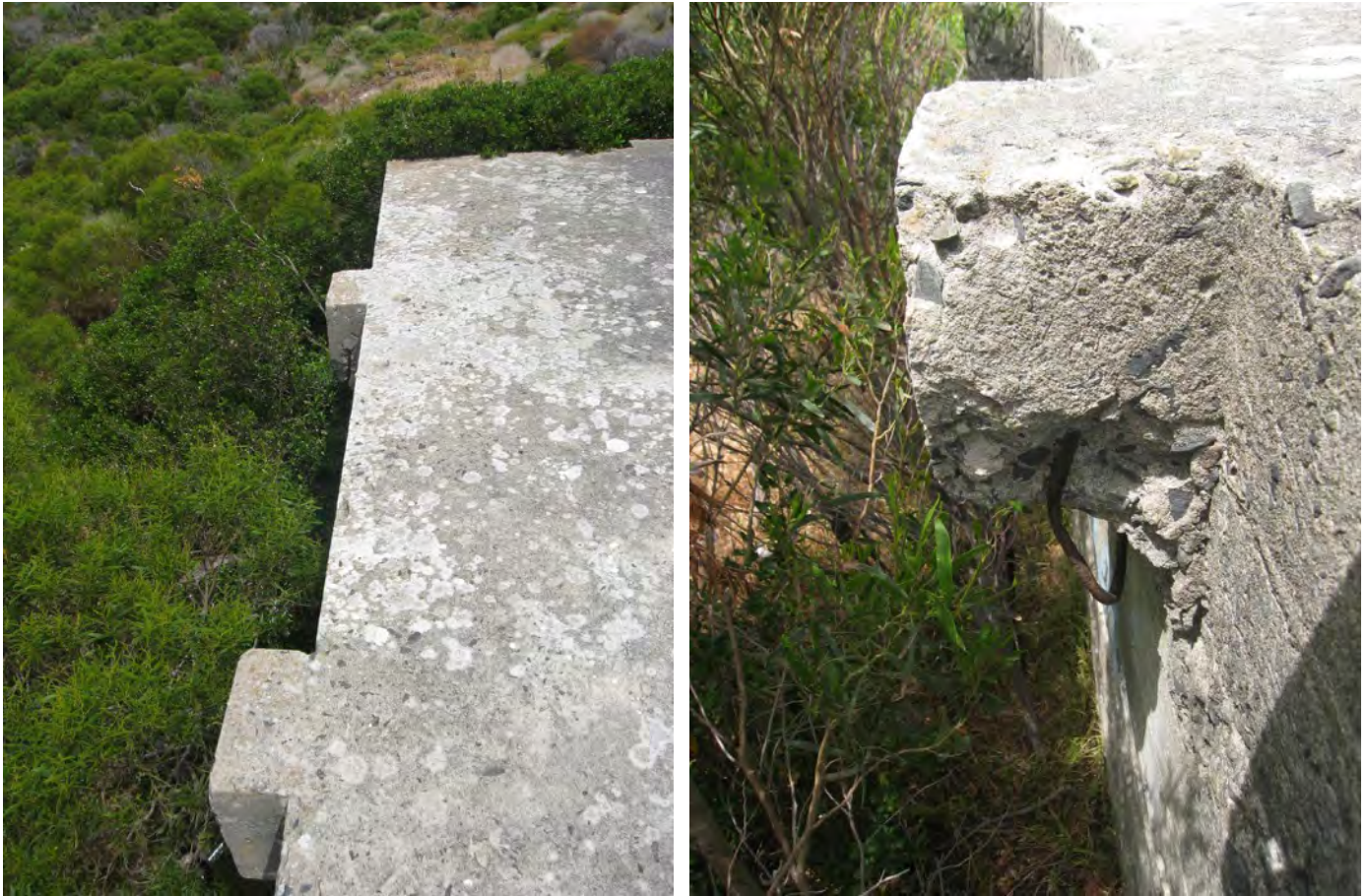
Figure 145: Ammunition Bunker No. 2 – Ventilation shafts
