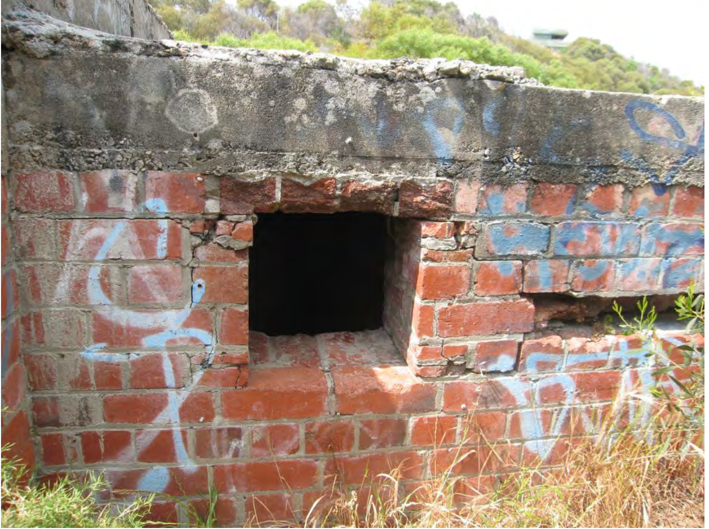
Figure 85: Operations Bunker – Openings in north wall
