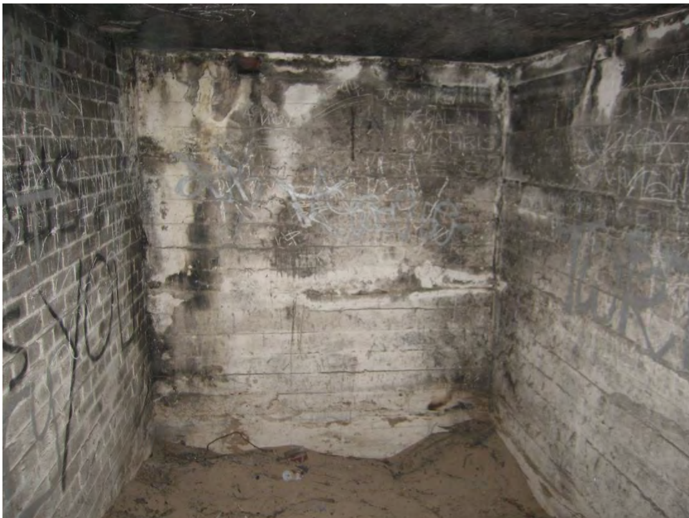
Figure 122: Ammunition Bunker – Room 1
