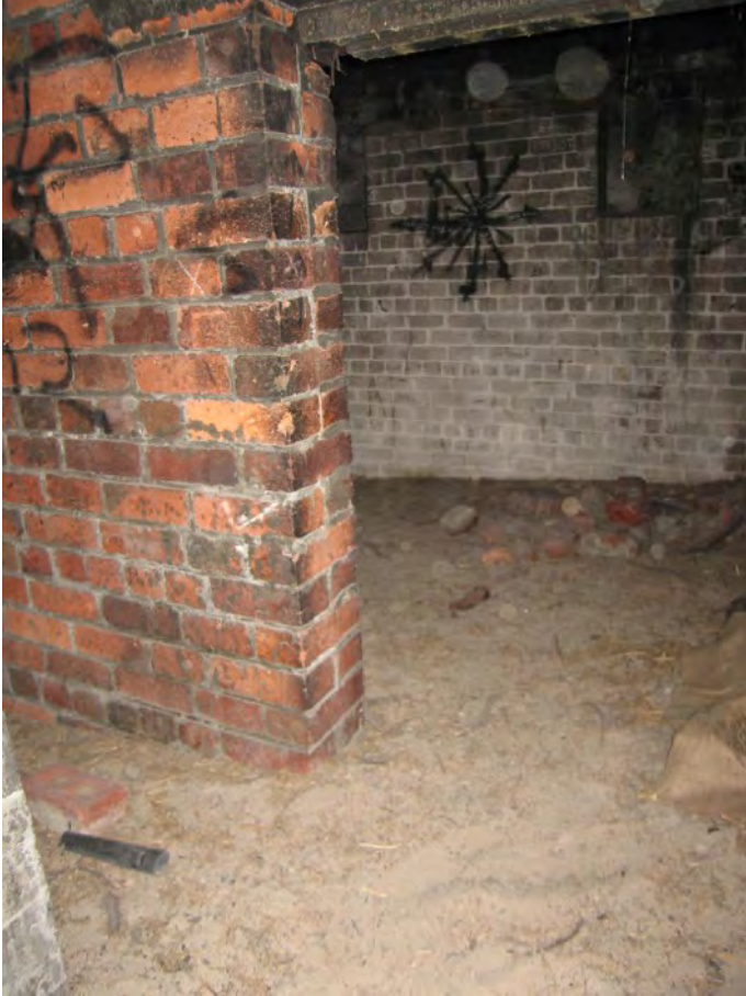
Figure 125: Ammunition Bunker – brick perimeter wall
