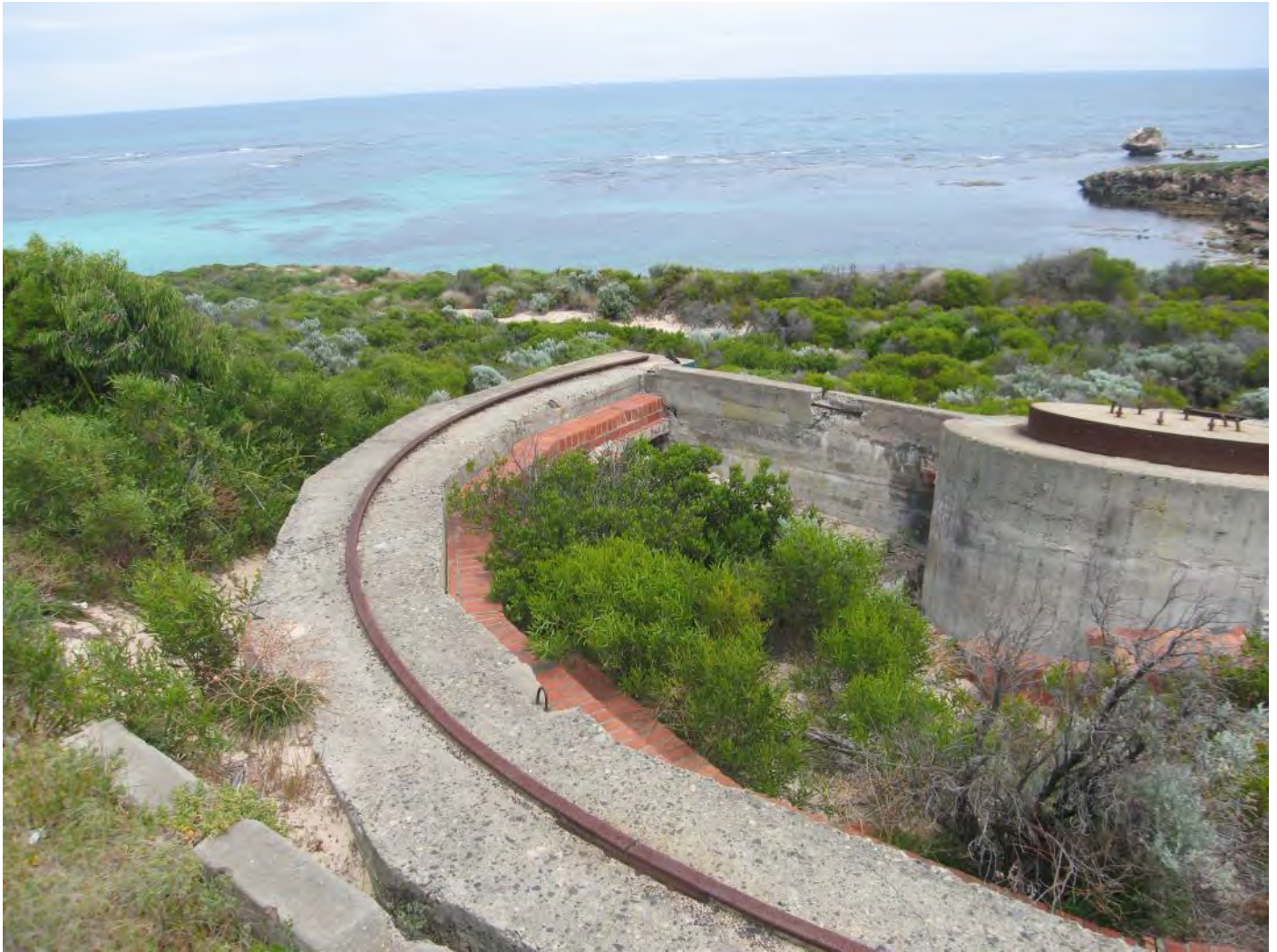
Figure 105: Gun Emplacement No. 1 – gun track
