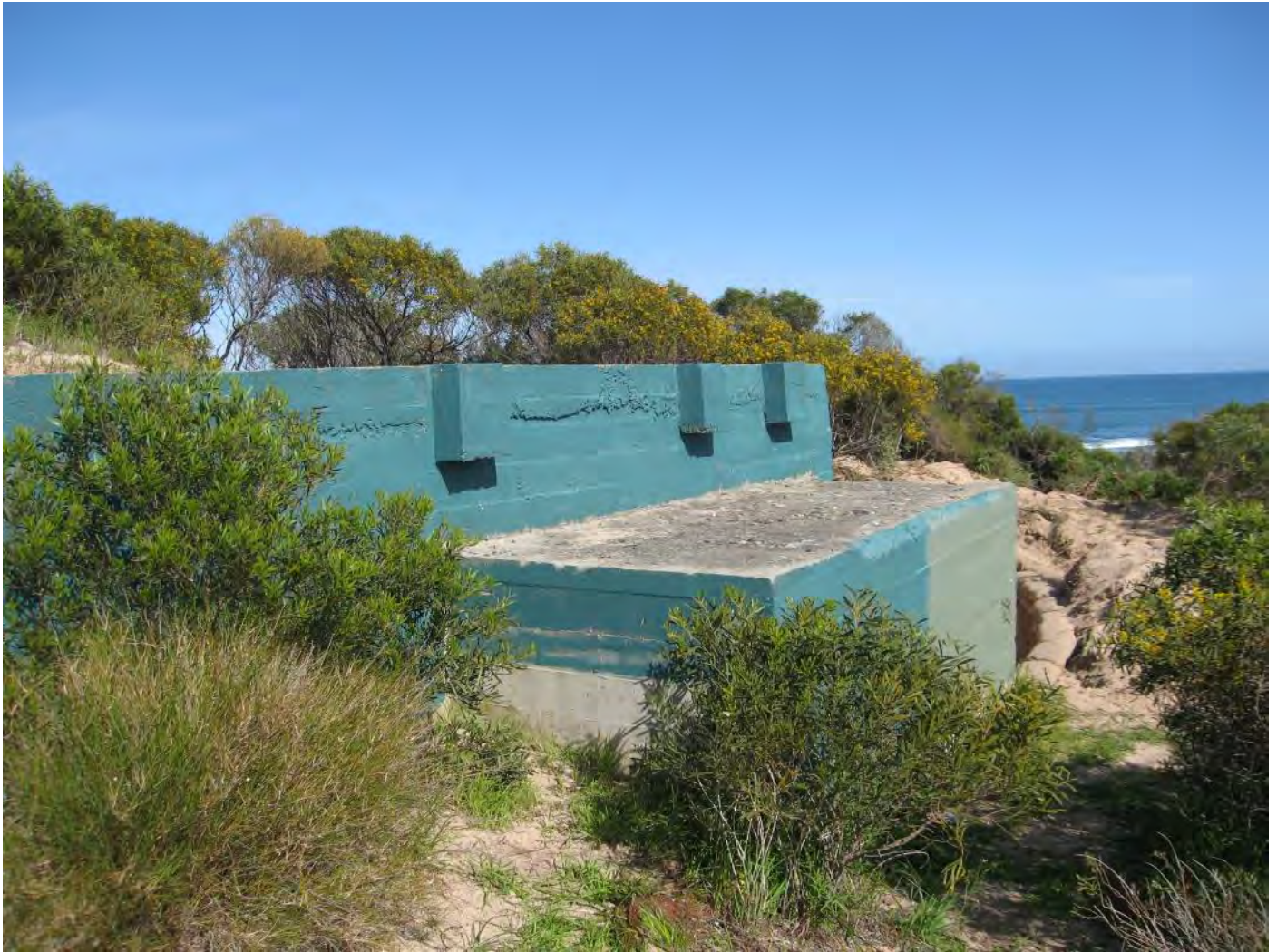
Figure 117: Ammunition Bunker – East elevation
