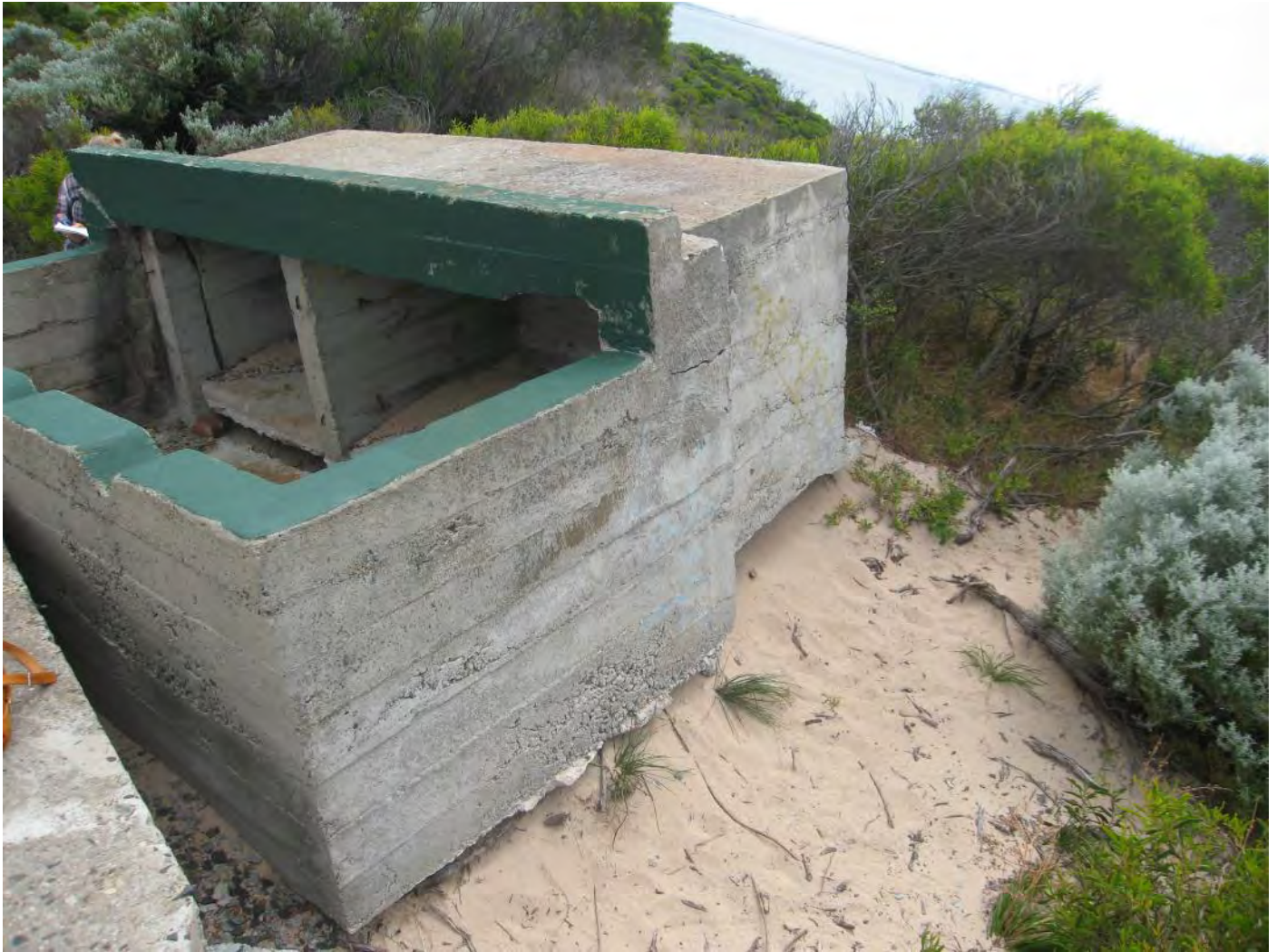
Figure 108: Gun Emplacement - Ammunition Store No. 1
