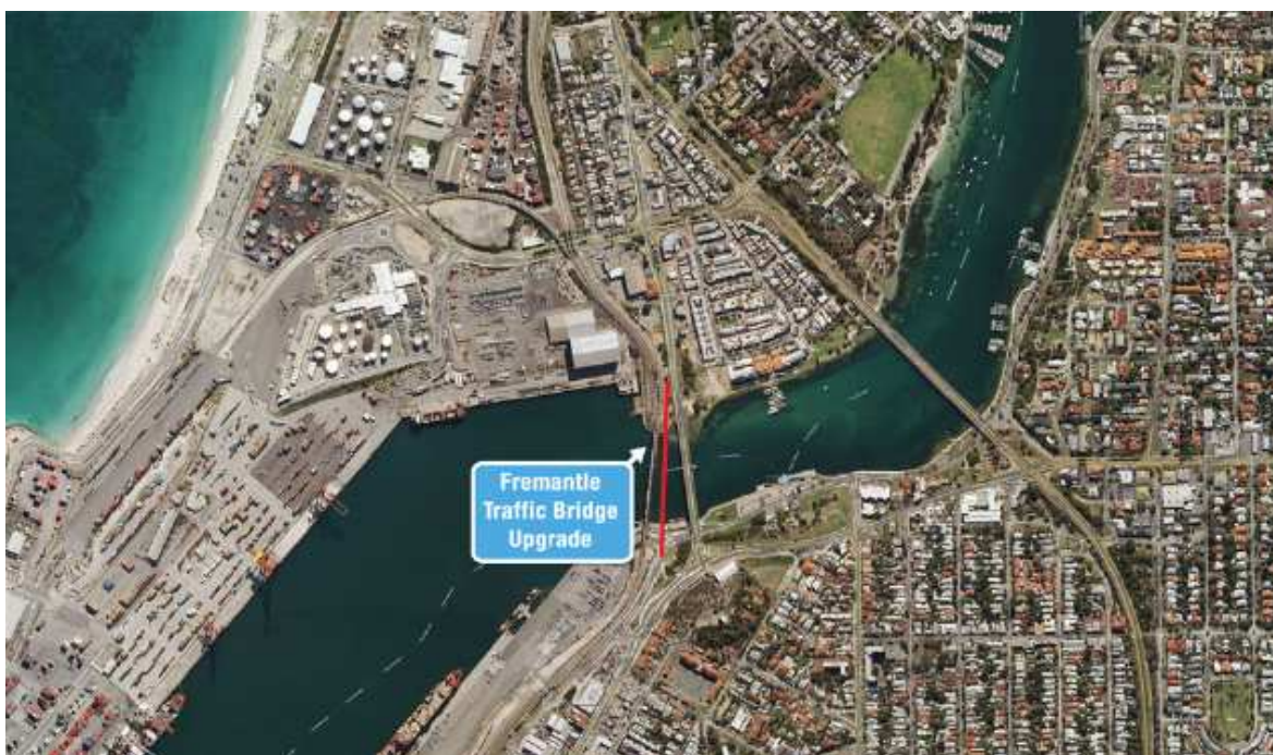
Figure 5: Upgrade of Fremantle Traffic Bridge
