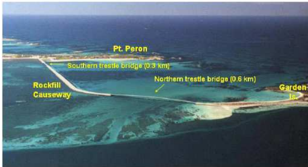
Figure 1. The Garden Island Causeway (looking south).
