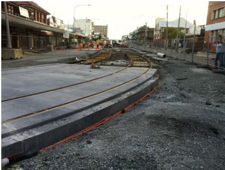
Light Rail track construction through South Port
