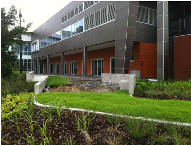
The GCUH Mental Health Wing has incorporated innovative design and security elements
