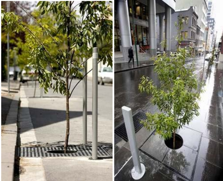
Water sensitive stormwater capture systems irrigate trees (above) and investment in stormwater harvesting (below) is increasing resilience to drying climate
