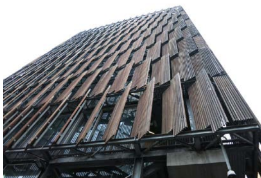
Automated solar louvers on the east facing side of CH2 adjust to solar activity
