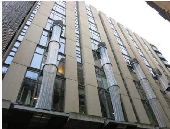
The tubes attached to CH2 capture rain water and provide ventilation
