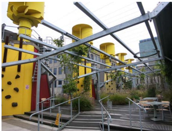
The rooftop garden is an inviting place for staff and also houses the wind turbines
