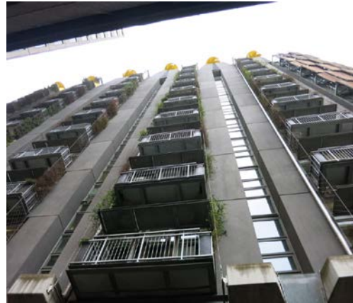
Balconies on south side of CH2 include plants to increase green space
