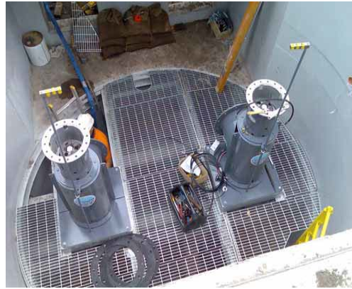
Stormwater pumping stations direct excess drainage and flood waters to the creek system
