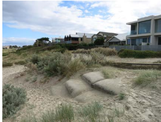
Sand bagging has been effective in stabilising and rehabilitating the dunes
