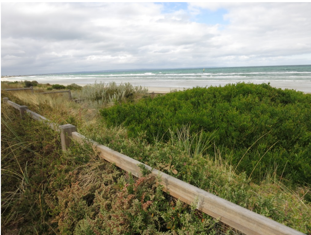
Vegetated retention basins along the North Aspendale foreshore have replaced pipe outfalls and treat and infiltrate stormwater runoff rather than direct discharge into the ocean
