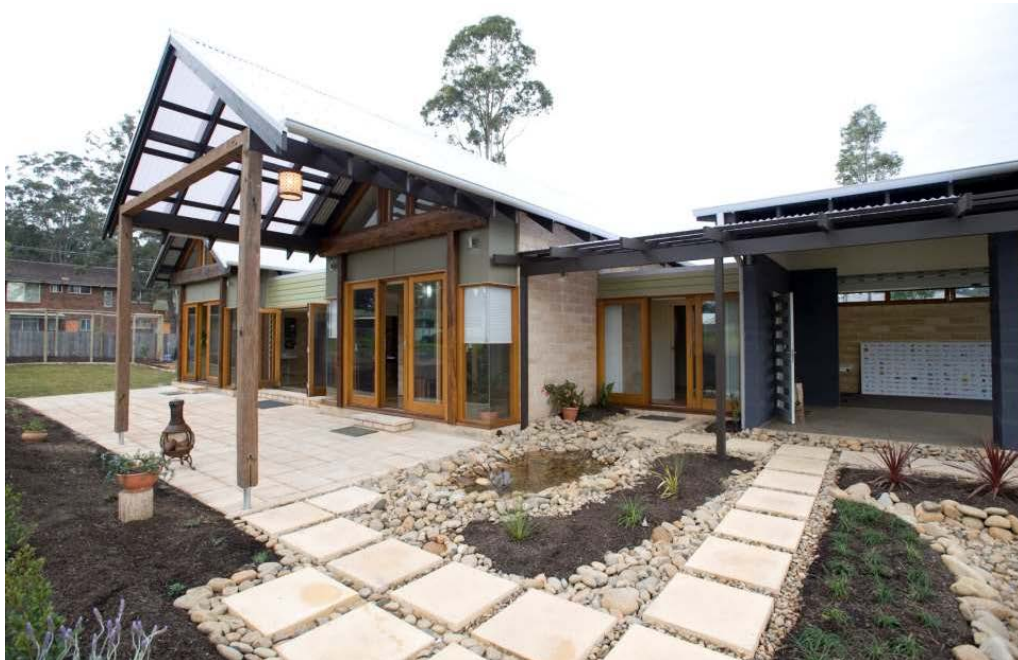
The Nowra sustainable house demonstration project has generated much community interest in sustainable design
