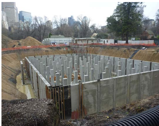
The underground storage tank, constructed wetland and water transfer pumping and storage system at Fitzroy Gardens ensures that the water quality is maintained for irrigation purposes
