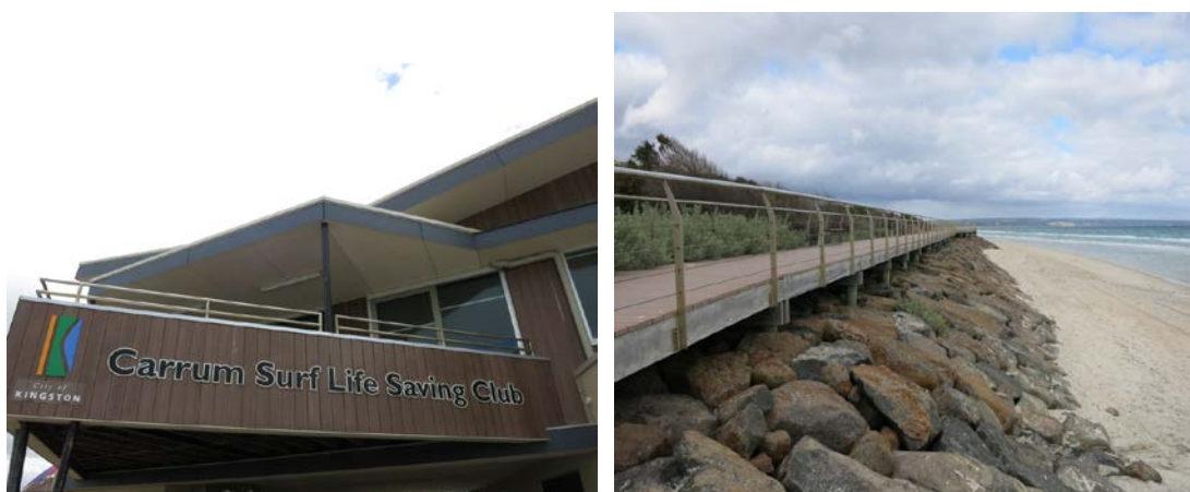
The Carrum Surf Life Saving Club is connected to the boardwalk and rock walling
