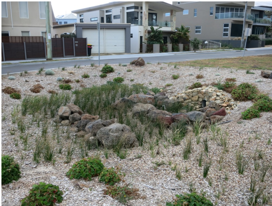
This vegetated infiltration basin replaced an ocean pipe outfall and was integrated into the redevelopment of a local park. The infiltration basin overflows to swale located behind the primary dunes to provide further infiltration in high flow conditions.
