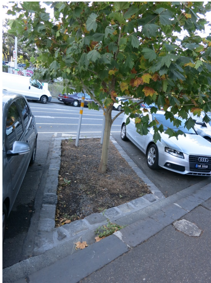
Simple and effective measures such as providing permeable areas surrounding street trees maximises infiltration and reduces compaction of tree roots
