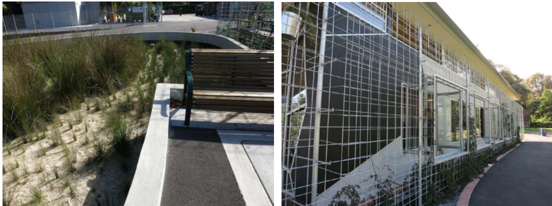
The vegetated wetland filter basin is located adjacent to the recently constructed visitor centre and café, which was built based on sustainability and energy efficiency principles
