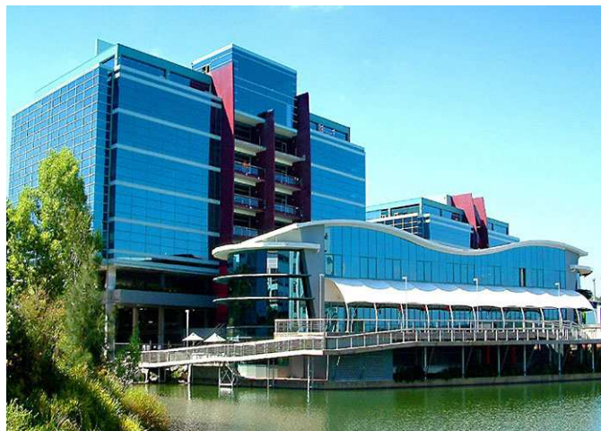
Quality buildings and landscaped gardens and open space are a key feature of the business park
