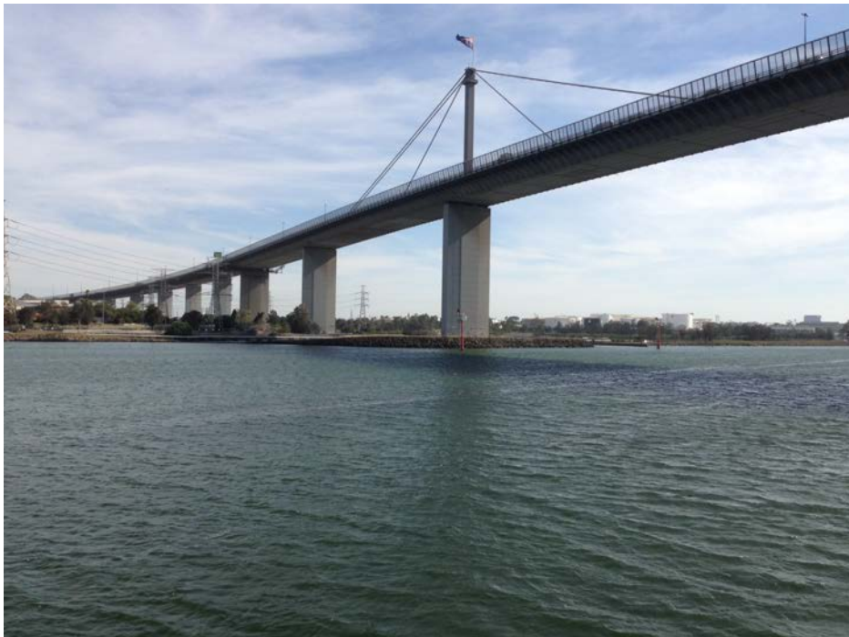
The Westgate Bridge looking north
