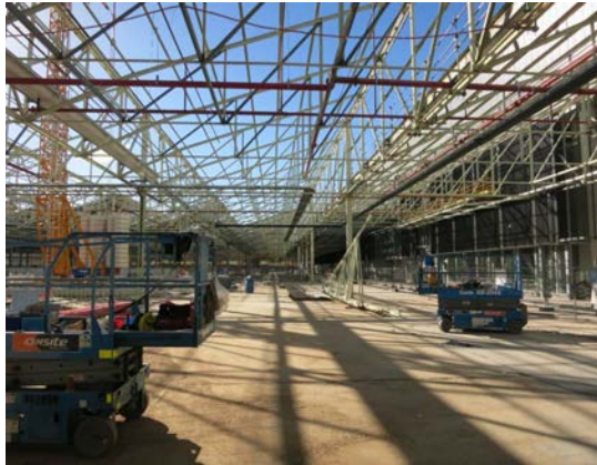
The steel construction shed structure has been retained and forms a key structural and design feature for Tonsley, with building constructed underneath the roof
