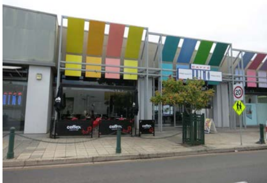
New shop fronts create street appeal
