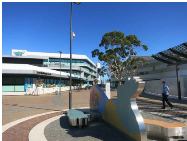
The SA Aquatic and Leisure Centre (right) is co-located with the GP Plus Health Care Centre (left), which offers a range of opportunities for synergies and shared services
