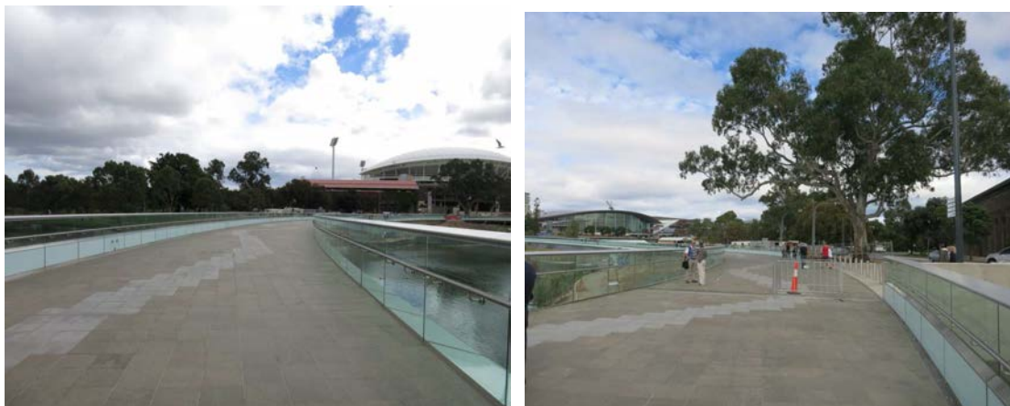
The Riverbank footbridge from the south bank looking toward the redeveloped Adelaide Oval (left) and from the north bank with the recently completed redevelopment stage of Convention Centre in the background
