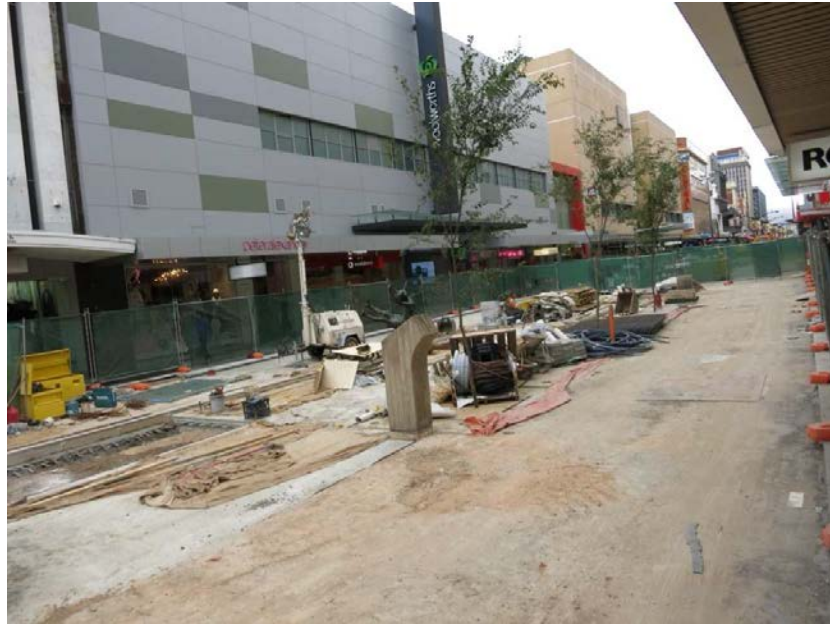
The second stage of the Rundle Mall redevelopment under construction
