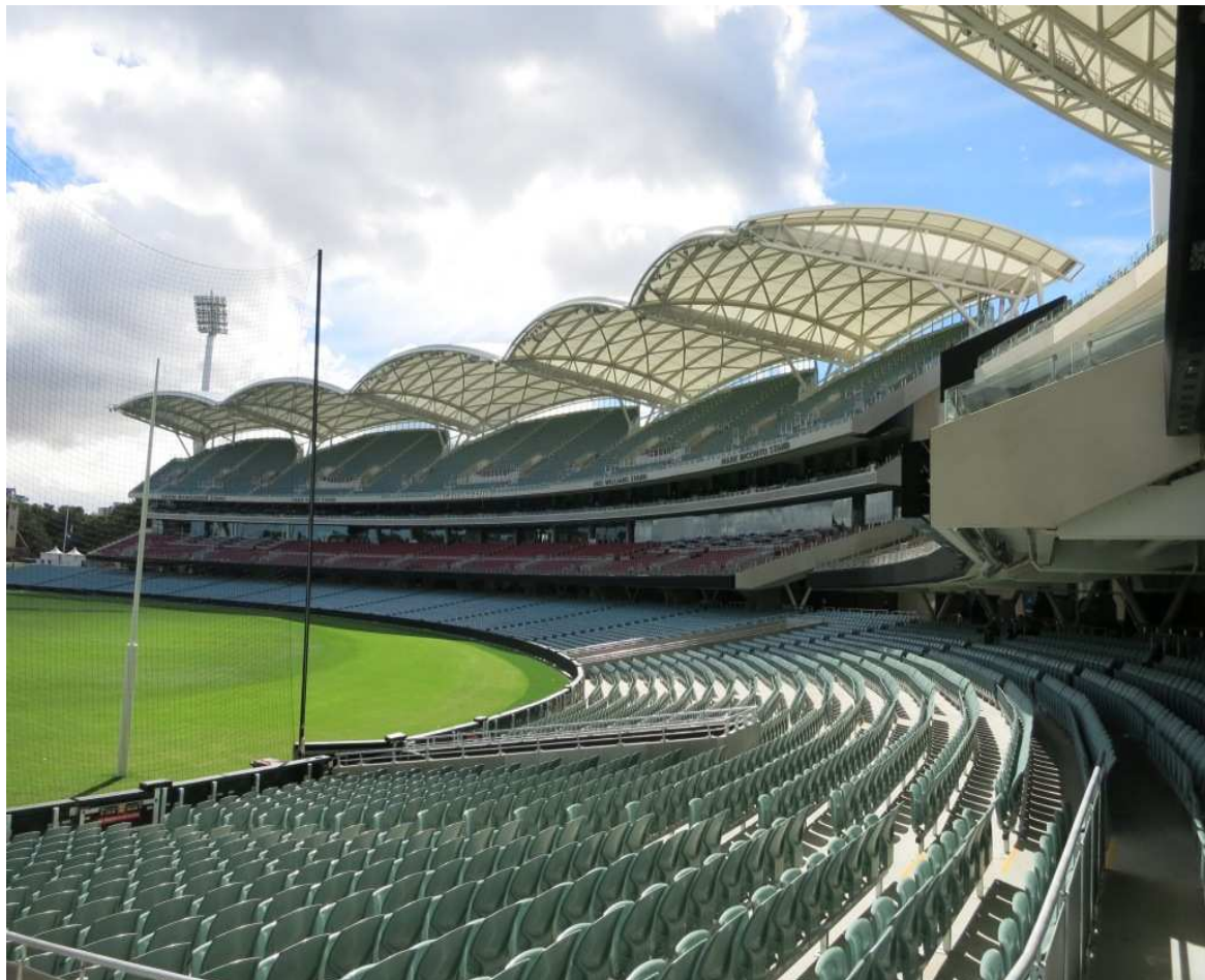
The eastern grandstands at the redeveloped Adelaide Oval uses a scalloped design that lets through light and breeze
