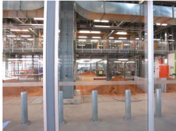
The steel construction shed structure has been retained and forms a key structural and design feature for Tonsley, with building constructed underneath the roof
