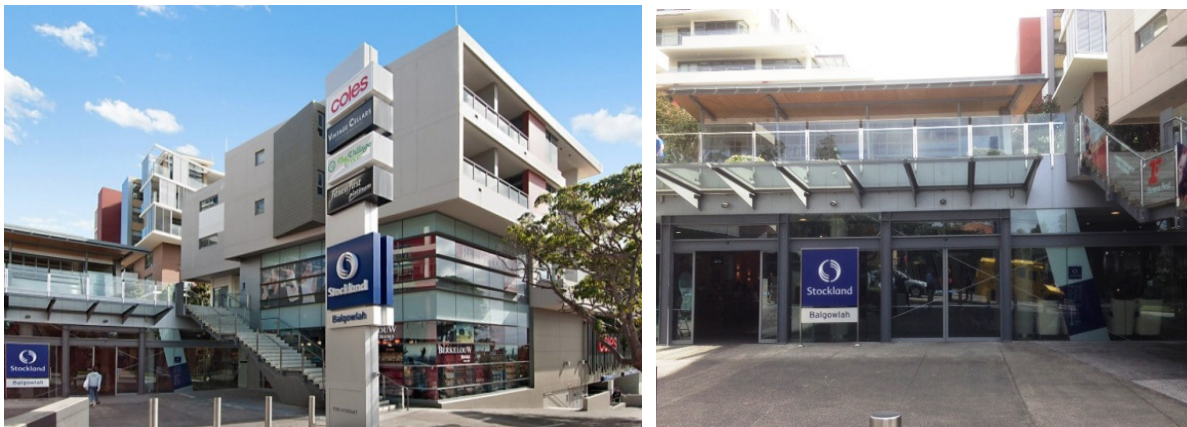
The Stockland Balgowlah development is a unique residential/retail precinct on Sydney's north Shore
