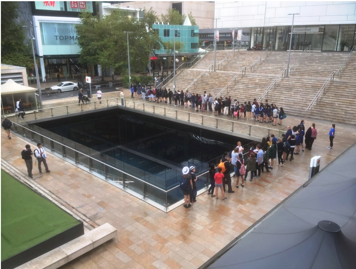
The Concert Hall and Theatre precinct has an underground library accessed from the main cultural centre plaza
