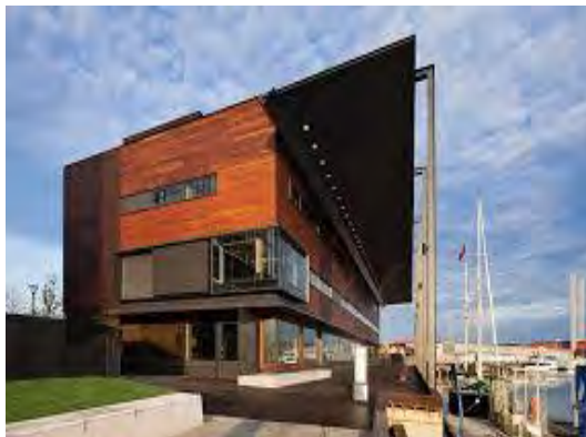
Library at the Dock uses sustainable laminated timbers as the main construction material
